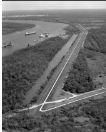
Marchand to Darrow levee on the Mississippi River, Louisiana.
