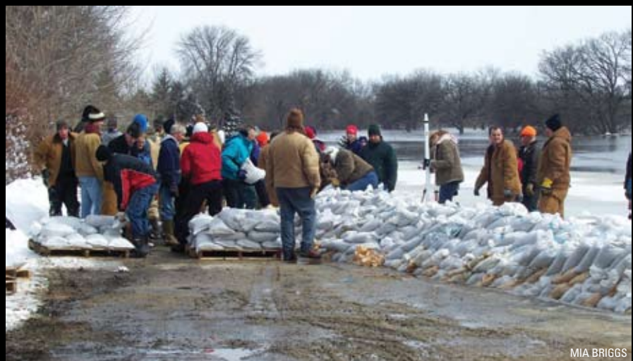
Top and above: A 45-foot-high dike protected the Fargo VA Medical Center from the 41-foot wall of water, but staff volunteered to sandbag the vulnerable north and south ends of the property.
