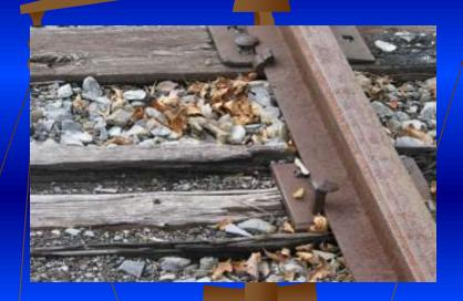
Because this rolling process was utilized, the rail has internal impurities, including slag, air pockets, and so on which makes the rail prone to breaks when heavy lateral forces are imposed; heavy cars like the ones proposed to transport the spent fuel rods would have an adverse effect on this size rail.
