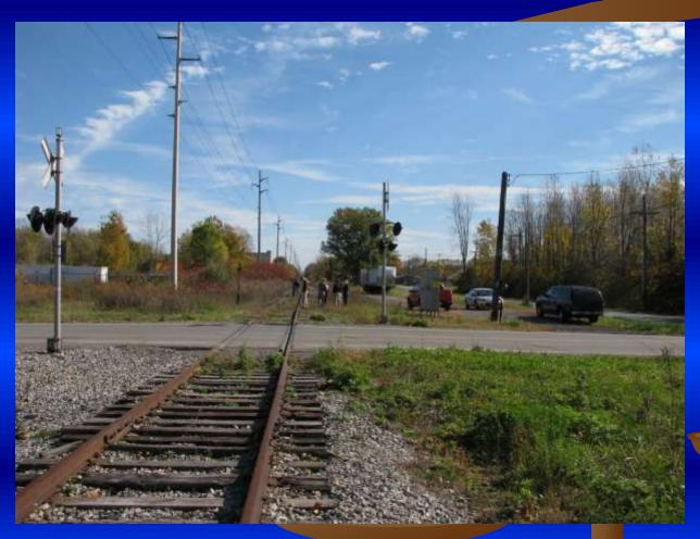
80 lb. Dudley rail on the Ontario Line (milled using the open hearth process in the early 1900s)
