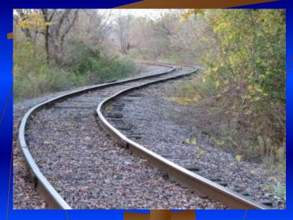
A series of S-curves between the CSX interchange and MP 18.0 on the Sodus Bay Line have sharp curves of 10, 11, 12, and 13 degrees. A curve greater than 8 degrees limits the type of rolling stock able to negotiate over them. A rigid frame triple axle truck could easily derail trying to negotiate these curves.
