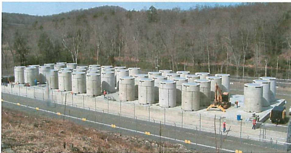
Figure 3. Independent Spent-Fuel Storage Installation
