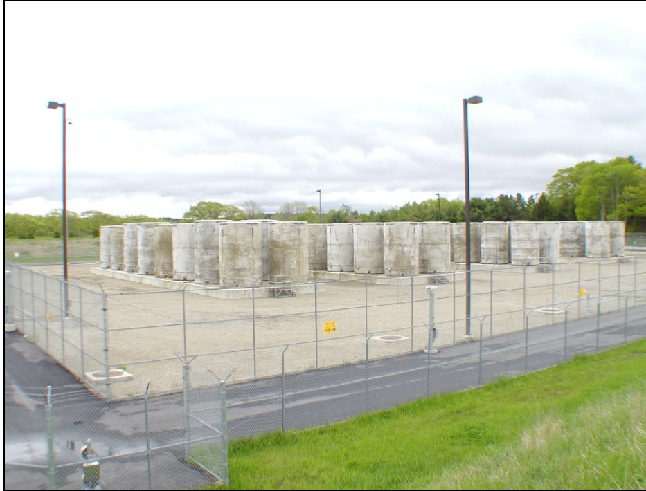
Figure 5. Dry Cask Storage Facility at the Decommissioned Maine Yankee Reactor Site
