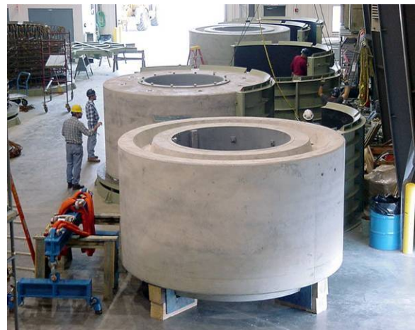
Figure 5-3 – Concrete Cask Construction
