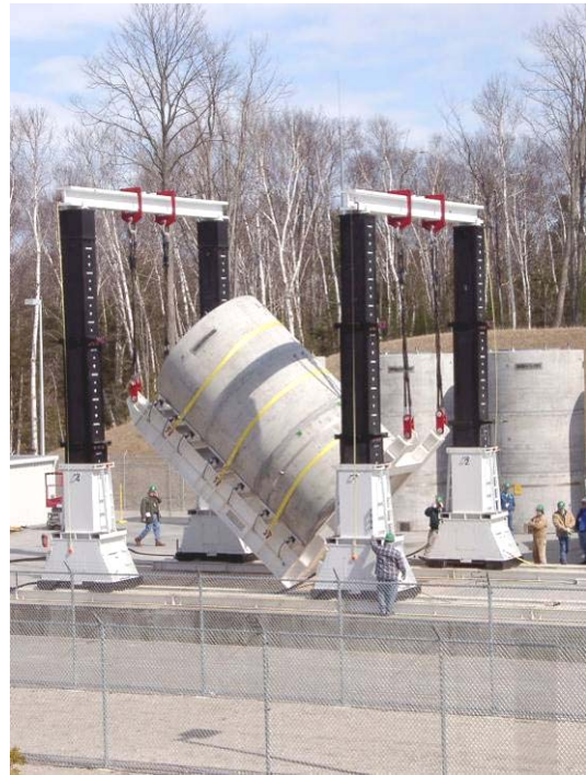
Figure 5-4 – Concrete Cask Handling
