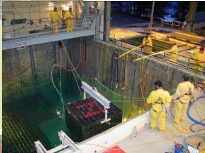
Removal of Spent Fuel Storage Racks from Spent Fuel Pool upon completion of fuel transfer to ISFSI -2004
