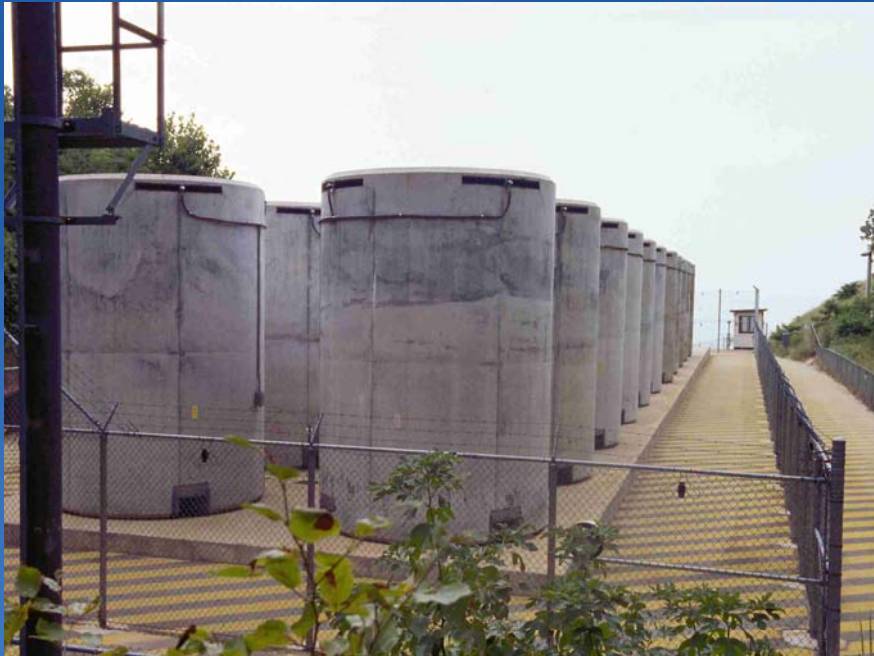
Vertical Storage Cask
