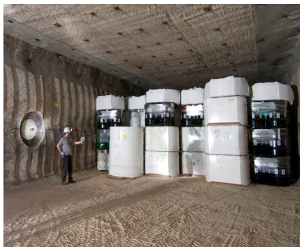
Fig. 3. Over 10,000 nuclear waste drums and standard waste boxes filling 1 of 56 rooms to be filled at WIPP over a 20-year period. Over 30 rooms have been filled as of September 2011. Note the high-activity remote handled waste (RH) plunged into boreholes in the wall to the right and plugged, while the contact handled waste (CH) fills the bulk of the room. The technician shown is receiving about a tenth of the radiation dose that we receive at the Earth's surface, ironic since he is standing in front of the nuclear waste.
