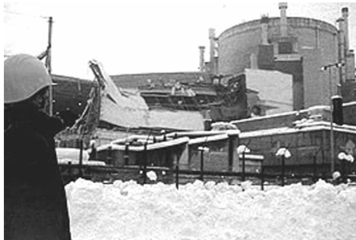
Figure 2.5 Superphénix collapsed turbine hall roof. Photo: Dissident-Media.
