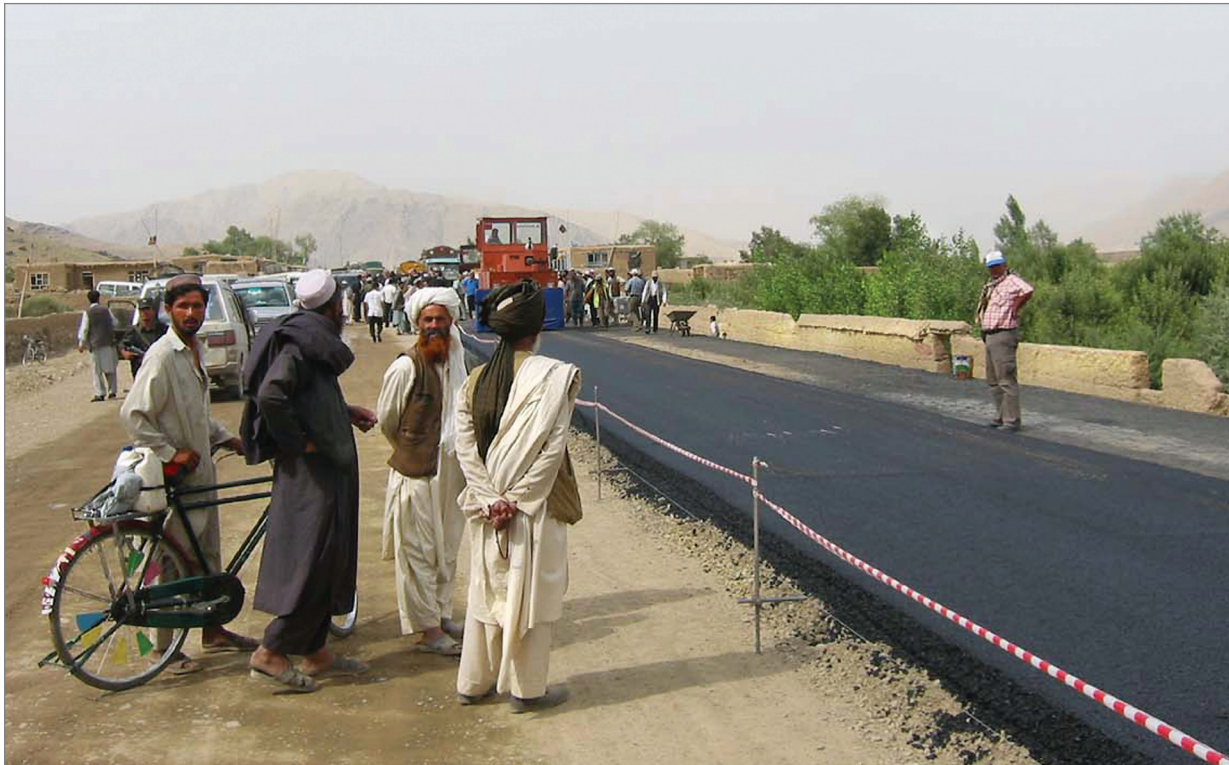
Kabul-to-Kandahar road construction, 2003. (USAID photo)
