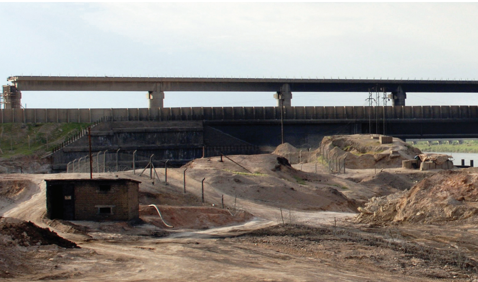
Al Fatah Bridge, with oil pipeline, after insurgent attack, Iraq , 2006. (U.S. Army photo)
