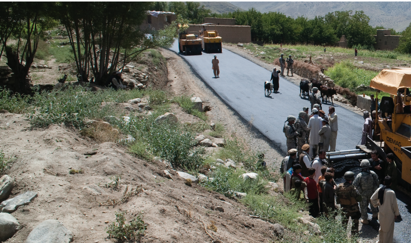
Road construction, Kapisa province, Afghanistan. (Defense photo)
