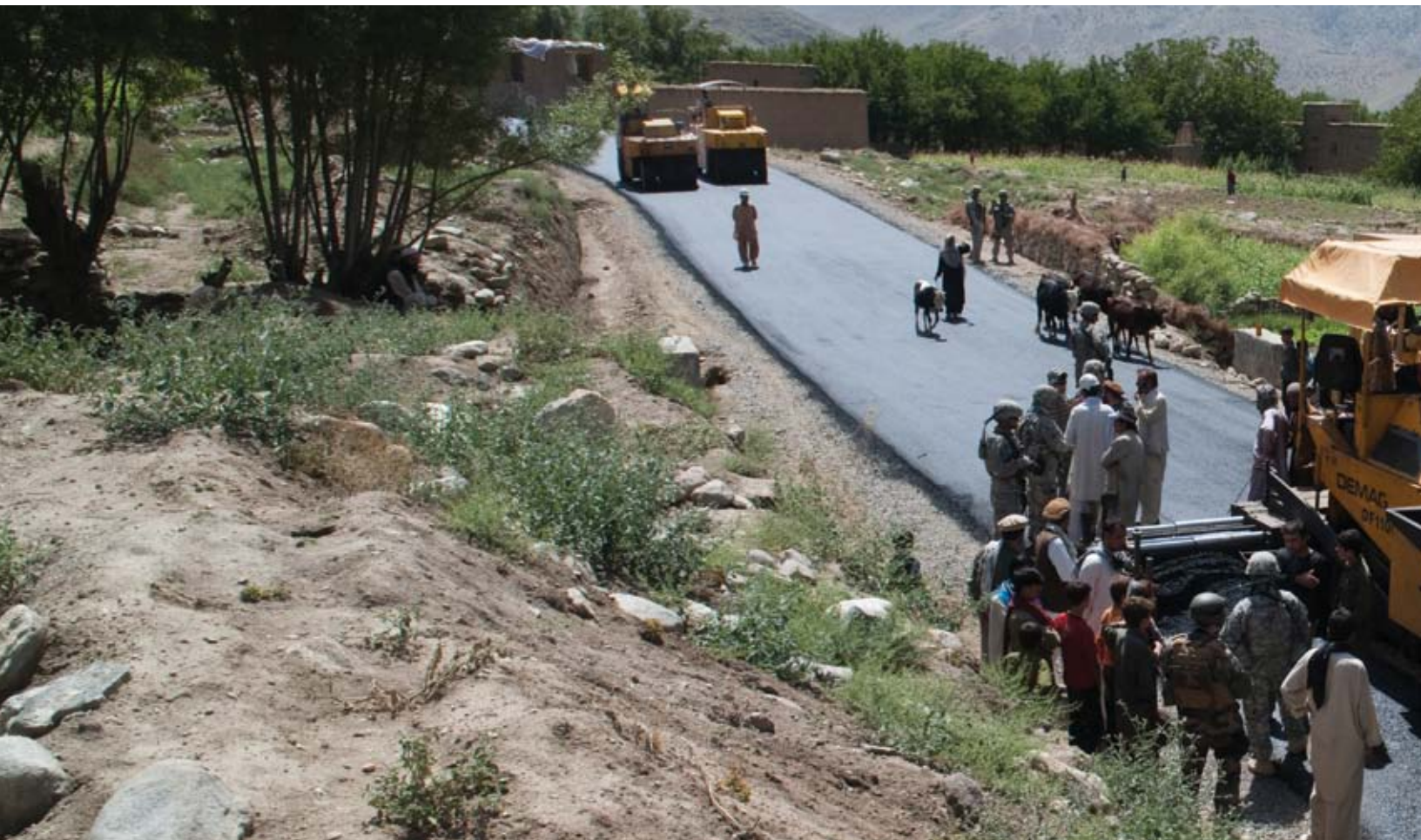
Road construction, Kapisa province, Afghanistan. (Defense photo)
