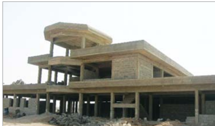
Kahn Bani Sa'ad Correctional Facility, Iraq, at the time of Parsons' termination, 2006. (U.S. Army Corps of Engineers photo)
