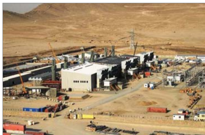
Kabul Power Plant, Afghanistan, 2010. (SIGAR photo)
