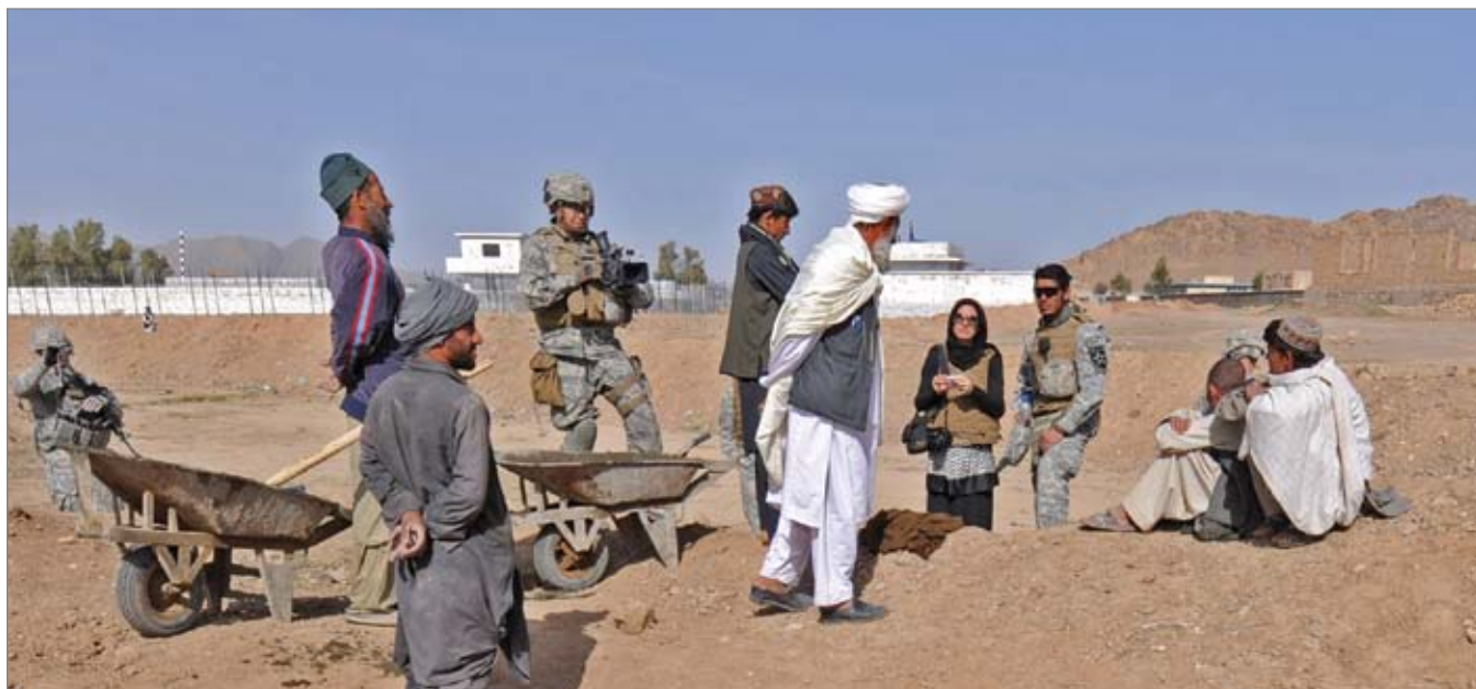
Afghan men working on USAID canal restoration project, Taktehpul, Afghanistan. (U.S. Air Force photo)
