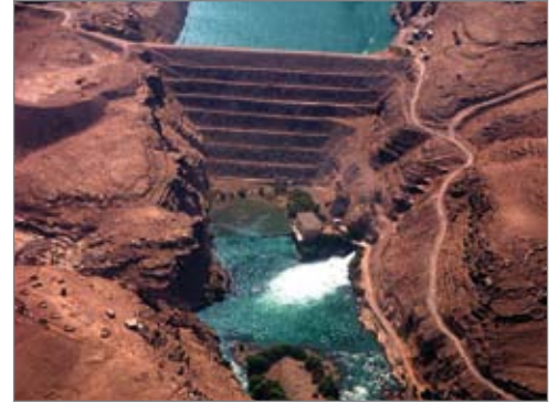
Kajaki Dam, Helmand Valley, Afghanistan, 2004. (U.S. Army photo)
