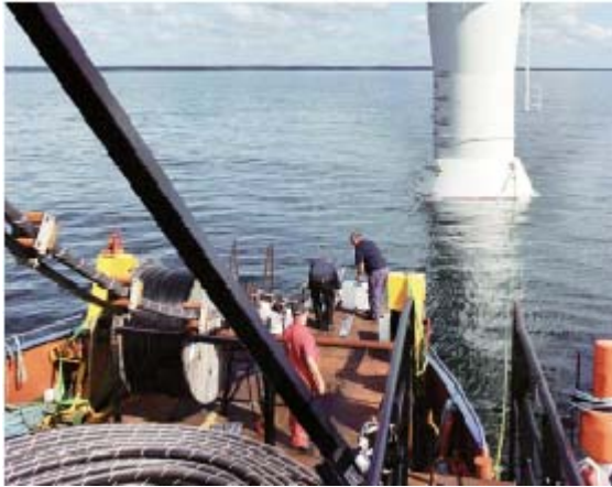
Figures 65: Cable deployment photos [Ref. 7.3].
