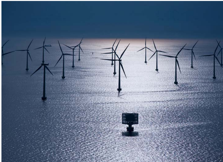
Figure 44. Lillgrund Sweden Transformer Station amid the Wind turbines.
