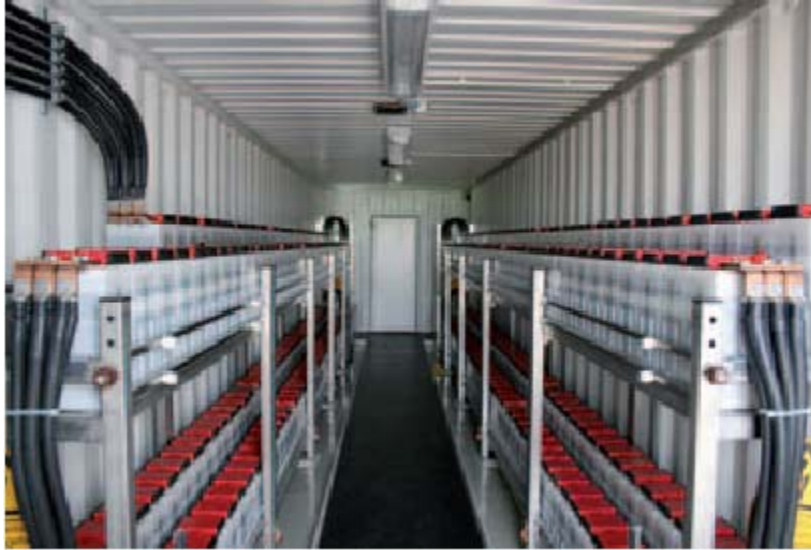
Figure 33 "The SAFT NiCd cells have a power capacity of 3000 kw for 2 minutes" [Ref. 3.15.1].
