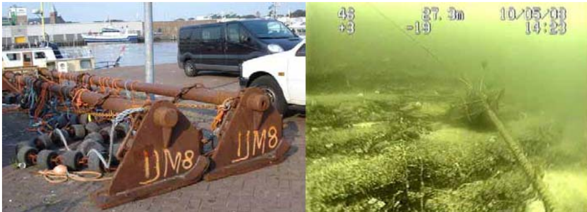
Figure 67: Clearing debris off the seabed
