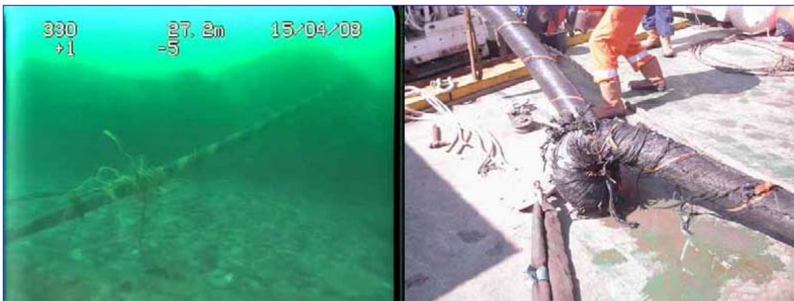
Figure 68: Ensuring there are no kinks in the line
