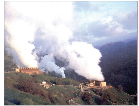
Geothermal power plant, CA
