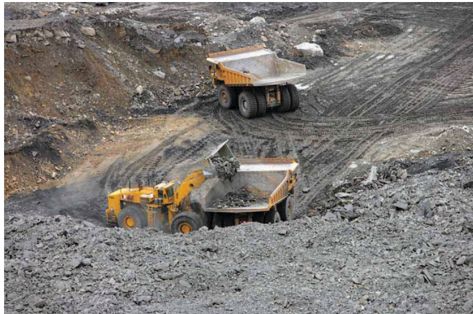
Blast overburden loaded into earth mover
