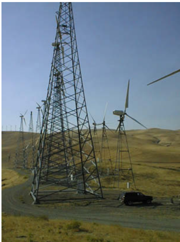
Photo 1-7. Example of a wind wall where 100-kW turbines are mounted on two different tower heights to catch a larger height domain of the wind. View is to the south.
