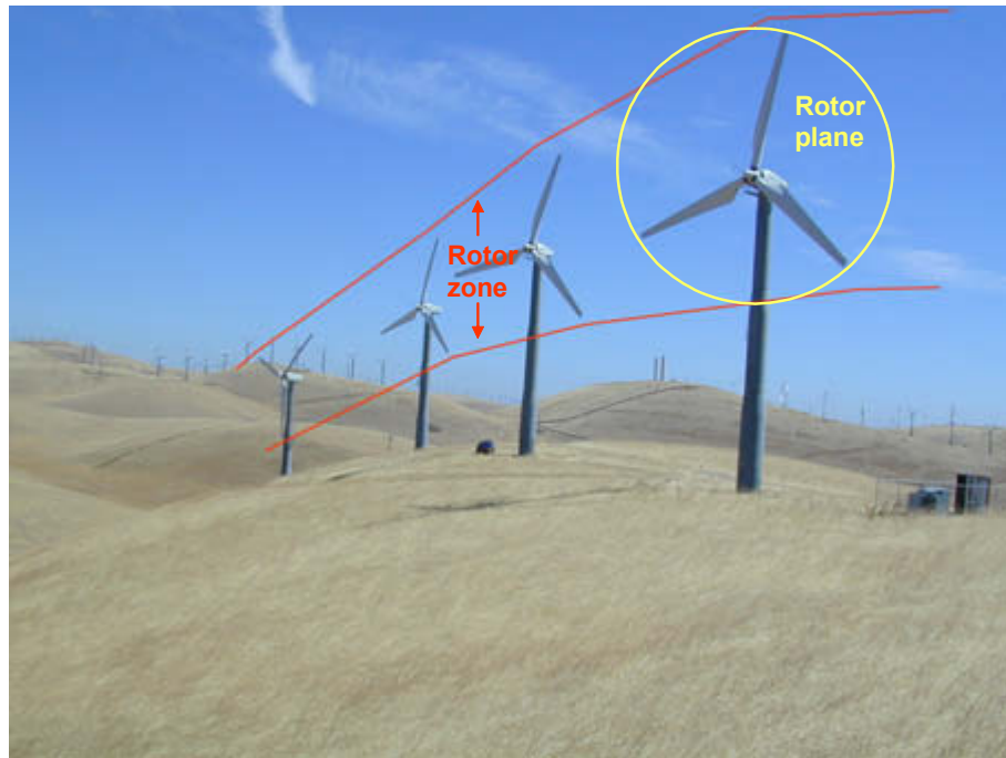
Figure 5-1. The rotor plane of a Bonus turbine and the upper and lower reaches of the rotor zone of a string of four turbines.
