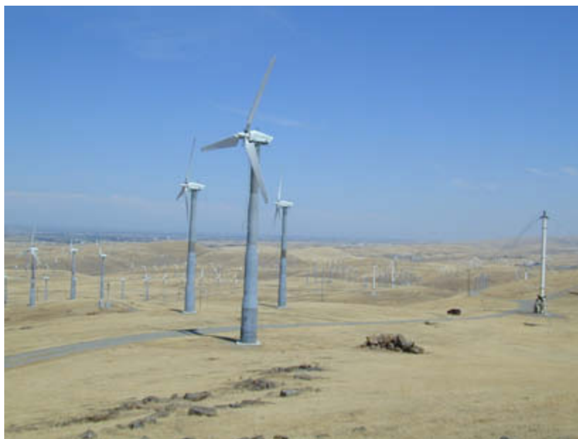
Photo 1-1. Bonus 150-kW wind turbines on tubular towers and Flowind 150-kW vertical-axis wind turbines on the right, view east.
