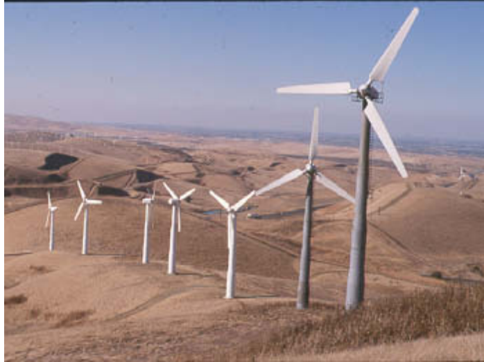
Photo 1-2. Bonus wind turbines in the foreground and Danwin 110-kW wind turbines downhill (white towers), view northeast.
