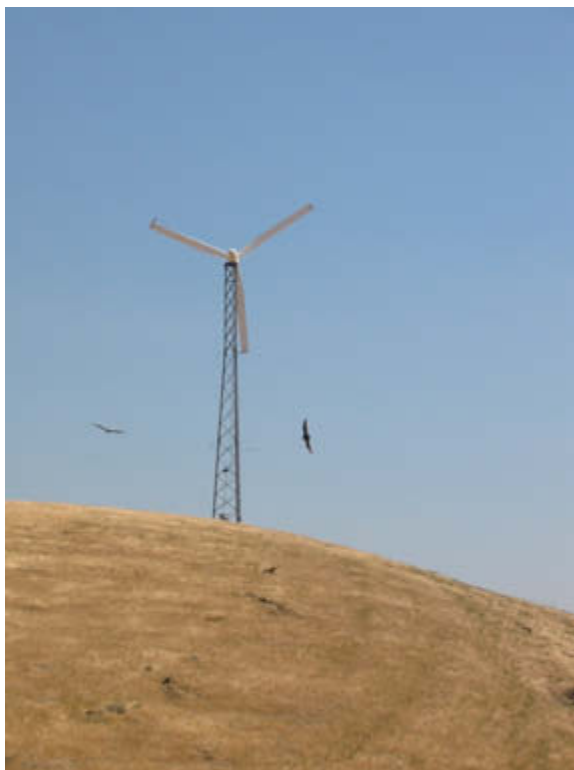
Photo 1-6. Enertech 40-kW wind turbine with two turkey vultures flying nearby.
