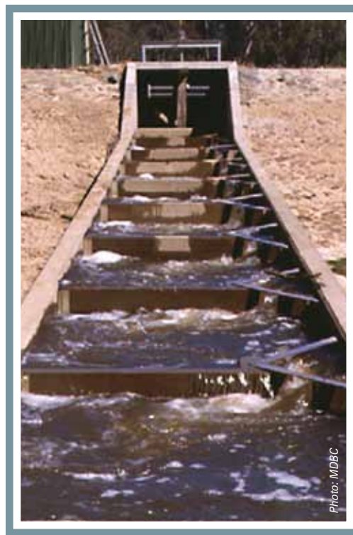
Fishway at Torrumbarry Weir on the Murray River
