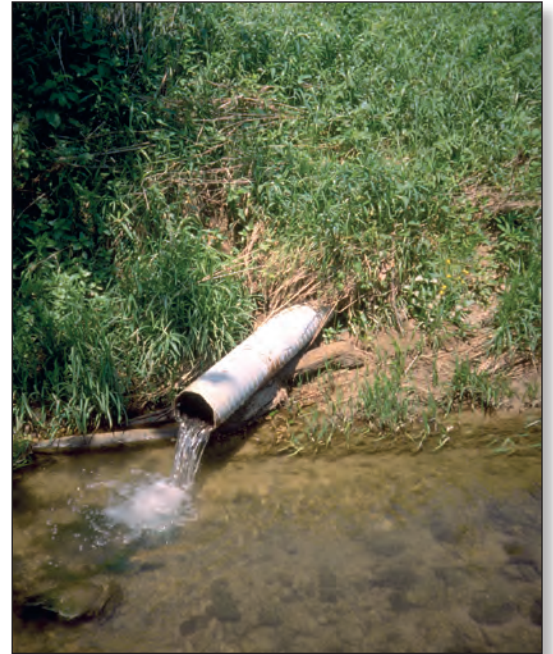
Tile drains buried at shallow depths reduce the water content of poorly drained soils and divert shallow groundwater to nearby streams. Photograph by Jeffrey Martin and Nancy Baker, U.S. Geological Survey.
