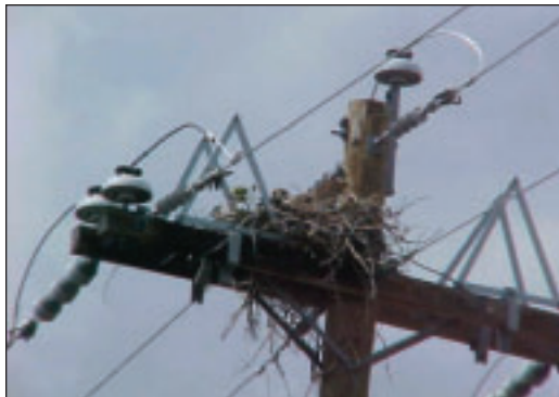
FIGURE 6.25: Red-tailed hawk nest on pole with triangle perch discouragers.
