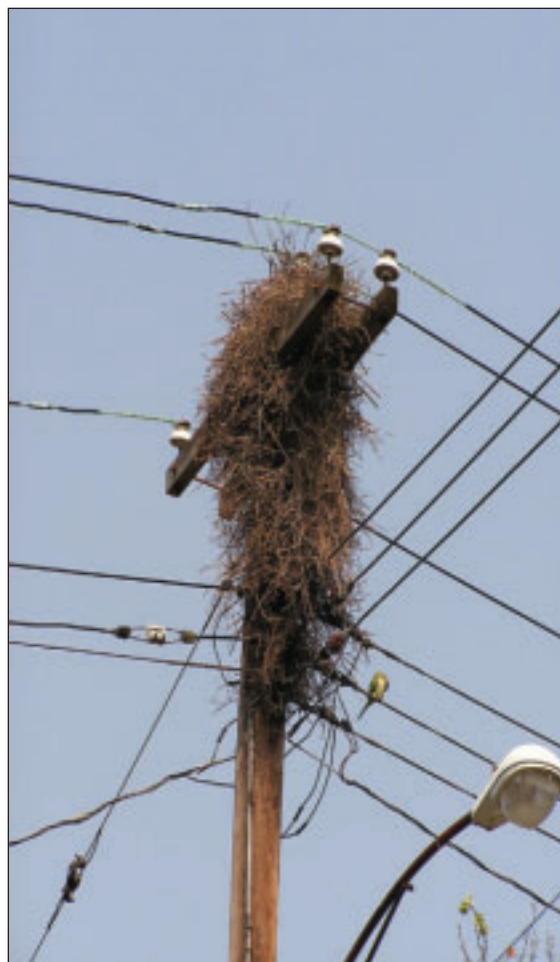
FIGURE 6.9: Monk parakeet nest on distribution pole.
