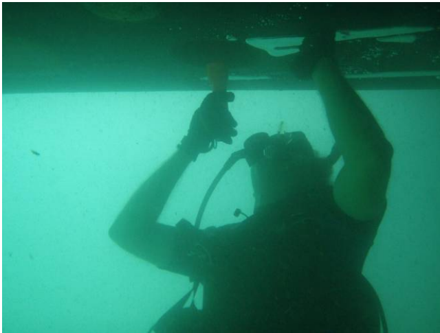
Inspection of a ship's hull.
