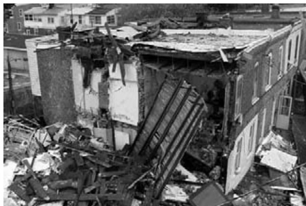
Damaged buildings on West Third Street in Wilmington, Delaware.
