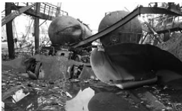
Rupture of railroad tank car in Freeport, Texas.
