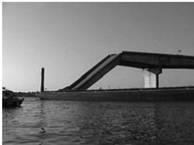
Damage to bridge following impact.
