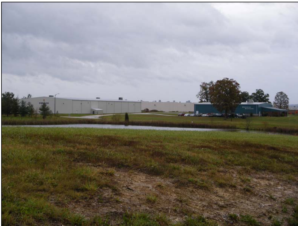
Morehead 801 Industrial Park
