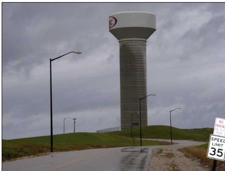
Morehead 801 Industrial Park Water Tank
