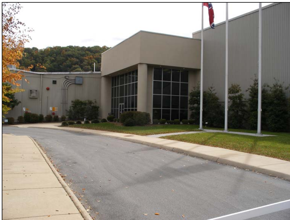
American Water Heater- Johnson City
