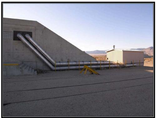
Plate 7.15 Typical earth-covered magazine modified with heating plant to create a constant temperature magazine (Courtesy U.S. Army, 2007)
