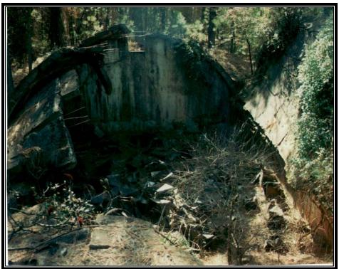
Plate 7.16 Igloo destroyed by detonation of contents, ca. 1955. Note how the force was directed upwards, even though the magazine was totally destroyed (Courtesy U.S. Army)
