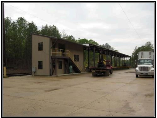
Plate 7.27 Typical explosives transfer building and loading dock showing enlarged office building and modified canopy over dock (Courtesy U.S. Army, 2007)
