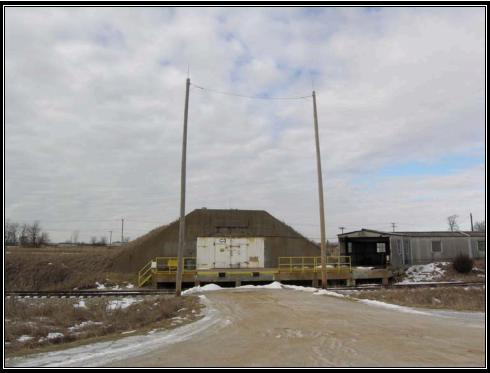
Plate 6.30 Typical shielding system of lightning protection at igloo storage (Courtesy U.S. Army, 2007)
