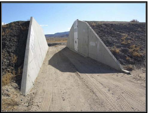
Plate 6.17 Typical concrete barricade opposite magazine entrance (Courtesy U.S. Army, 2007)
