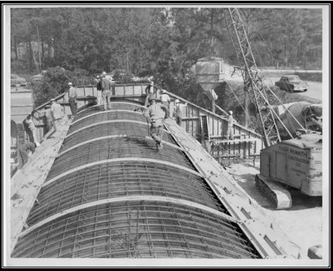
Plate 7.17 Construction of igloo magazines, ca. 1953. Note welder moving across top of arch (Courtesy U.S. Army)
