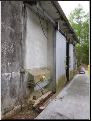
Plate 7.29 Sliding doors of typical Stradley magazine (Courtesy U.S. Army, 2007)
