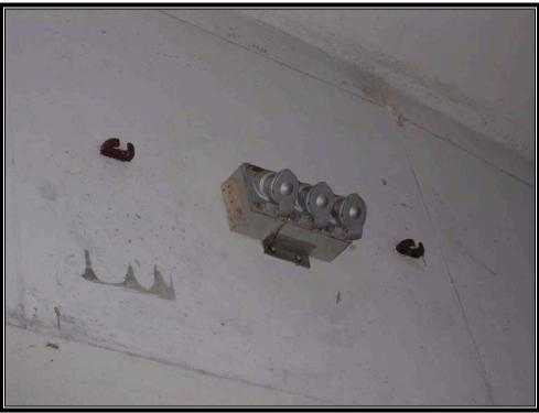
Plate 6.31 Typical explosion-proof electrical connection on interior of igloo. A similar plug on the exterior was connected to a portable generator when electricity was needed inside the magazine (Courtesy U.S. Army, 2007)
