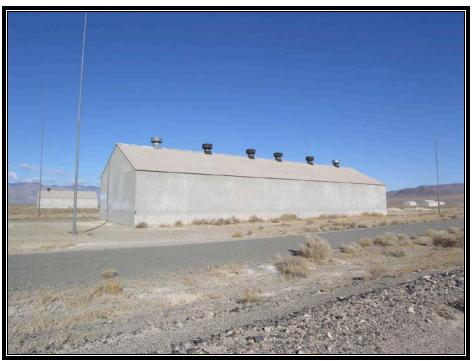
Plate 6.29 Typical group lightning protection for aboveground magazines (Courtesy U.S. Army, 2007)
