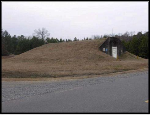
Plate 6.34 Typical igloo storage with truncated walls of the Huntsville type (Courtesy U.S. Army, 2007)
