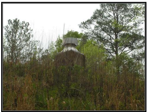
Plate 7.31 Ventilator at rear of typical Stradley magazine (Courtesy U.S. Army, 2007)
