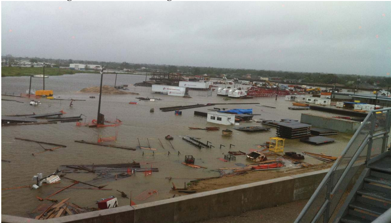
Figure 4. Seabrook site flooded during Tropical Storm Lee September 3, 2011.
