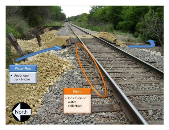
**Figure 5.** Photo shows storm water debris on the track, near the open deck bridge (0.1 mile west of the accident site). Water flow under open deck bridge is also indicated as flowing in southeast direction.
