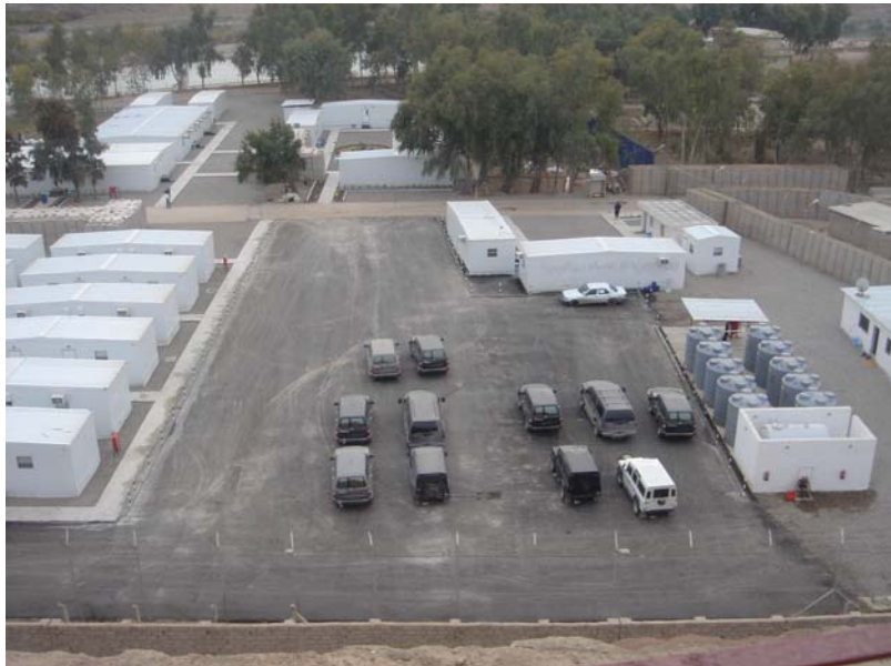
Photo 4. This photo, taken December 11, 2004, shows a portion of the secured encampment installed at the Mansuria Project site. Billeting trailers are on the left, water storage tanks on the right, construction administration and support facilities in the background; security wall in the upper right, and security/support vehicles in the foreground.
