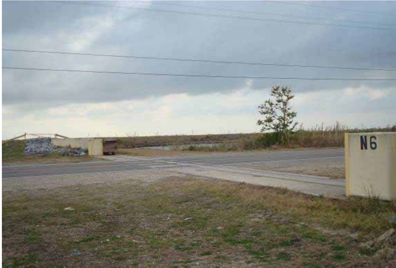
Photograph 8. US 11 Floodwall and Floodgate at LPV 109
