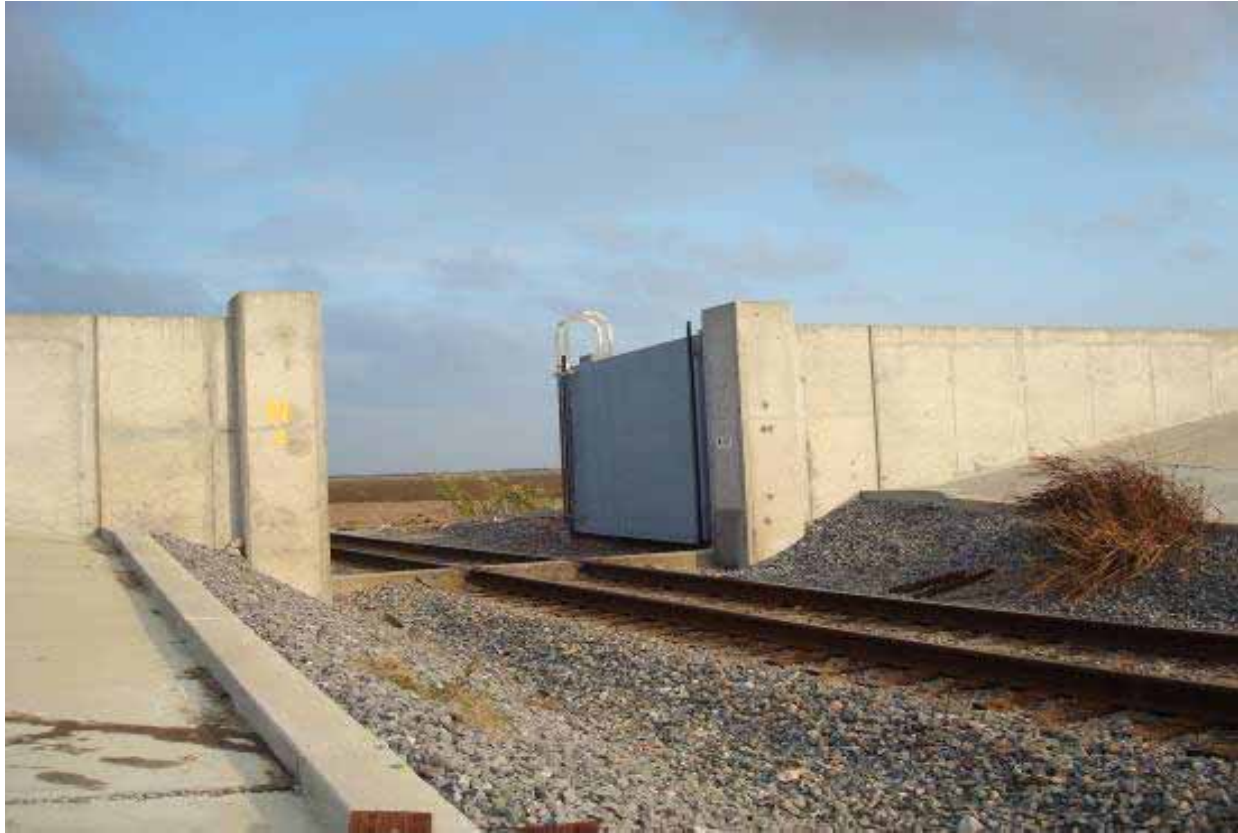
Photograph 2. Floodwall, Floodgate and CSX Railroad at LPV 110
