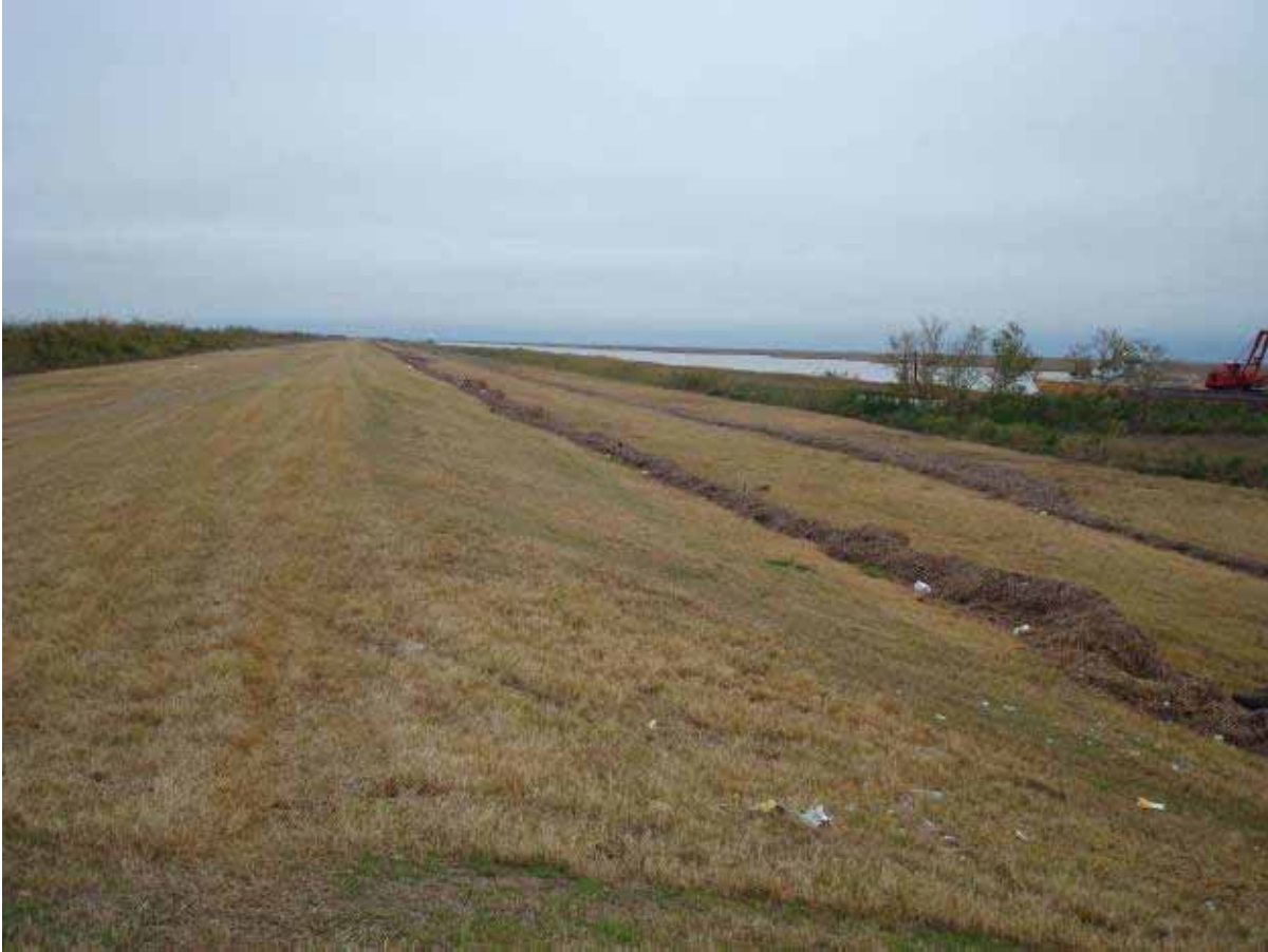
Photograph 3. LPV 111 Levee Adjacent to the GIWW
