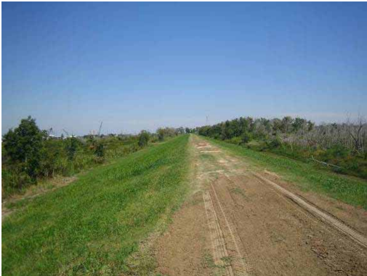
Photograph 1. LPV 109 Levee; Photograph Taken Looking South
