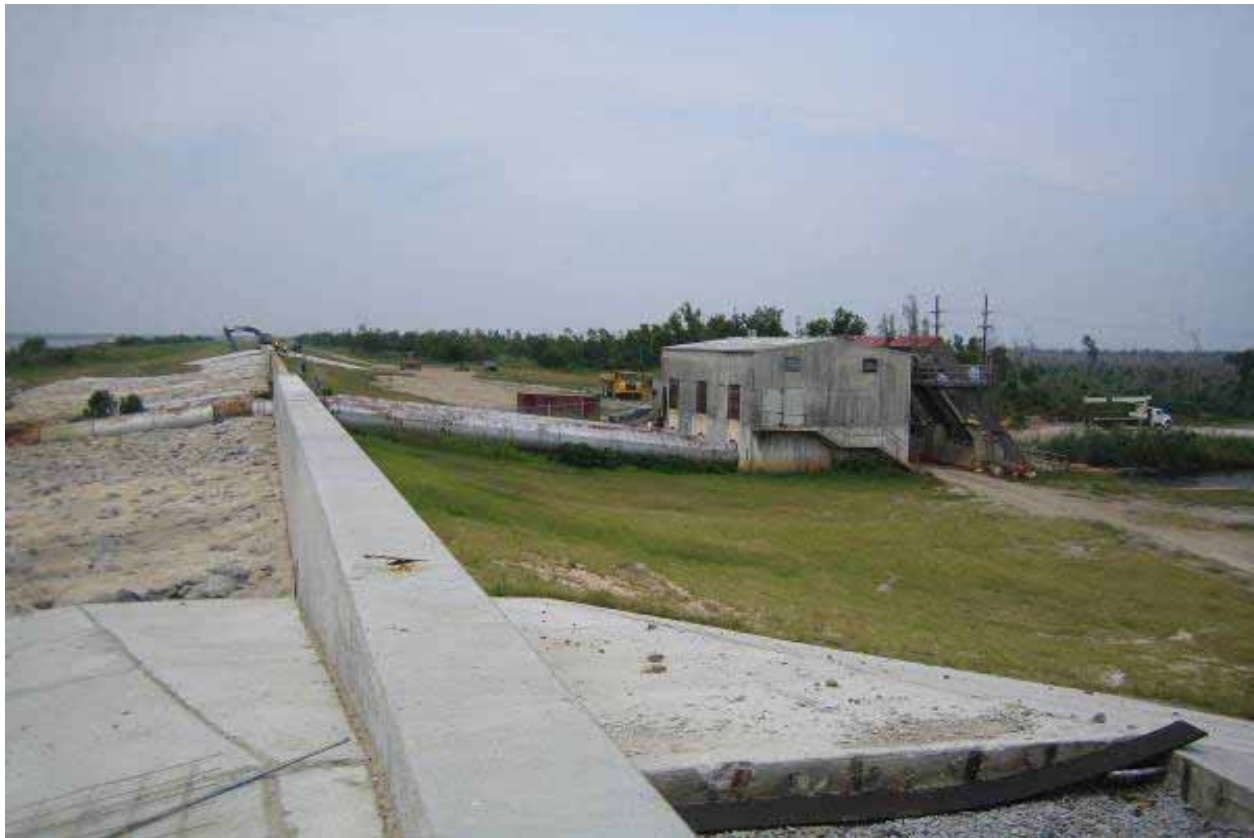
Photograph 5. T-wall and Pump Station No. 15 at LPV 111; Photograph Taken Looking West towards Paris Road
