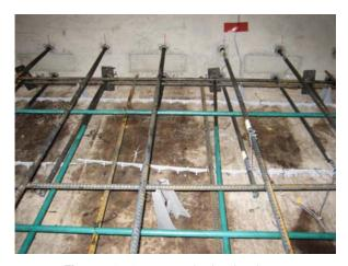
Figure 9-4 – Form savers for dowel anchorage.
