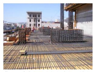
Figure 9-6 – Conflict between the location of collector reinforcing with a nonstructural component.
