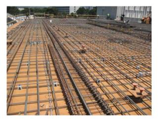
Figure 9-2 - A long collector with confinement reinforcement.
