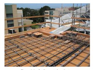
Figure 9-3 – Confinement of a collector.
