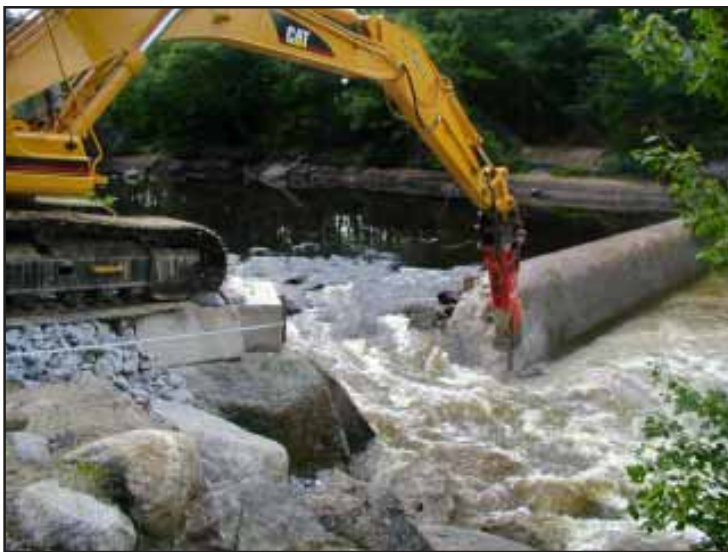
The Henniker Dam was breached to allow American eels and other migratory fish to reach habitat that had been blocked for nearly 100 years by this dam on Contoocook River in New Hampshire.
