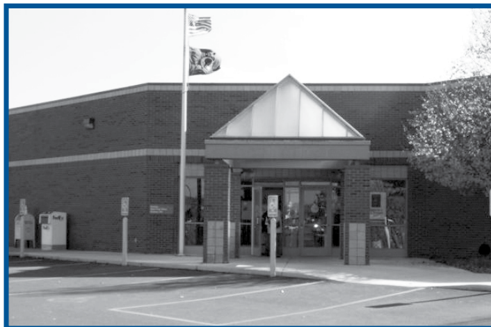
A valid business case existed for consolidating mail processing operations from the Beckley, WV, Post Office (pictured) into the Charleston, WV, P&DC.
