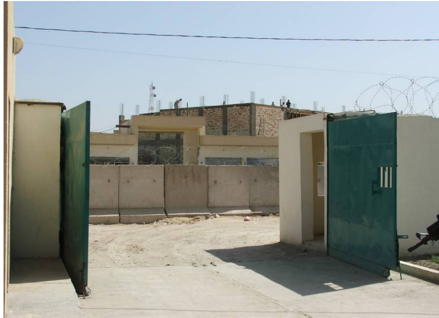
Site Photo 2. Main Entry Gate
