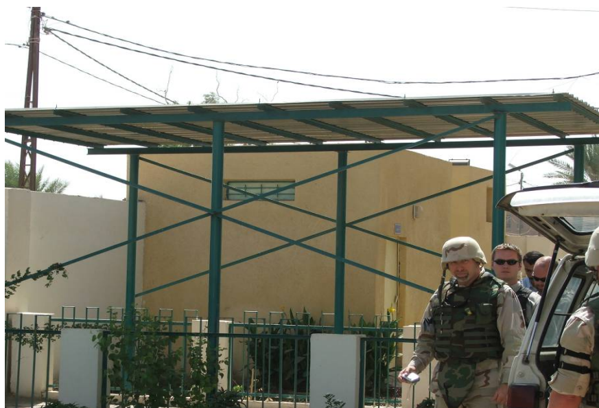
Site Photo 6. Entrance Canopy
