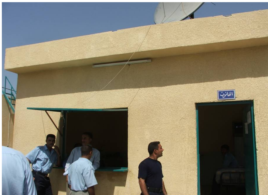
Site Photo 8. Exterior View of the Cafeteria Building
