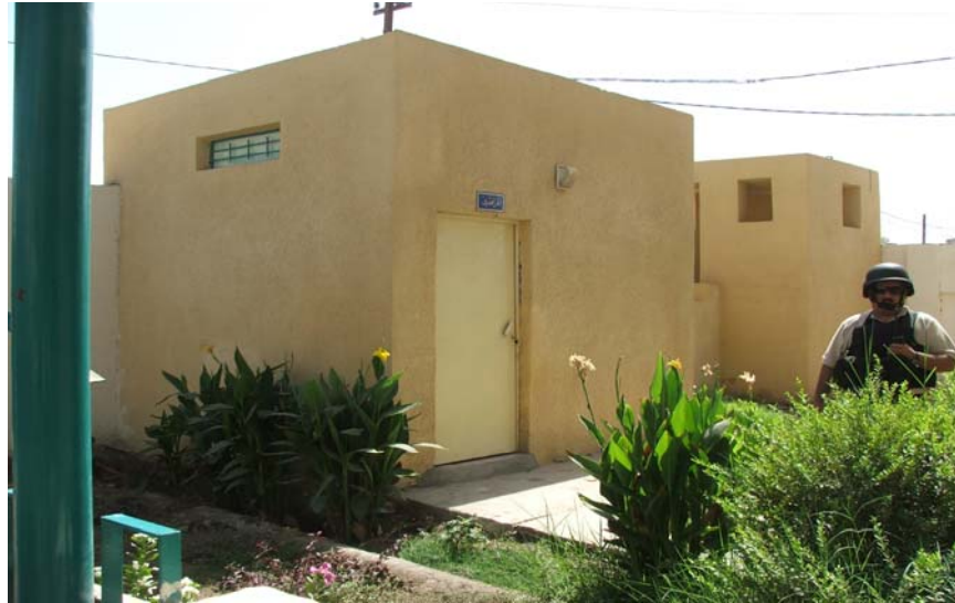
Site Photo 9. Exterior View of the Information Building
