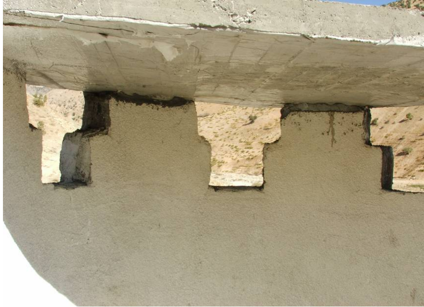
Site Photo 17. Parapet Corner Turret on Roof (Safrah #634 Border Post)
