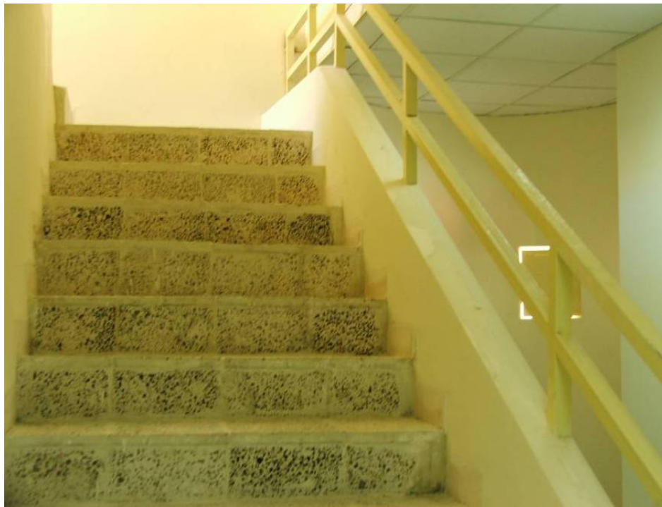
Site Photo 14. Interior Stairwell (Safrah #634 Border Post)
