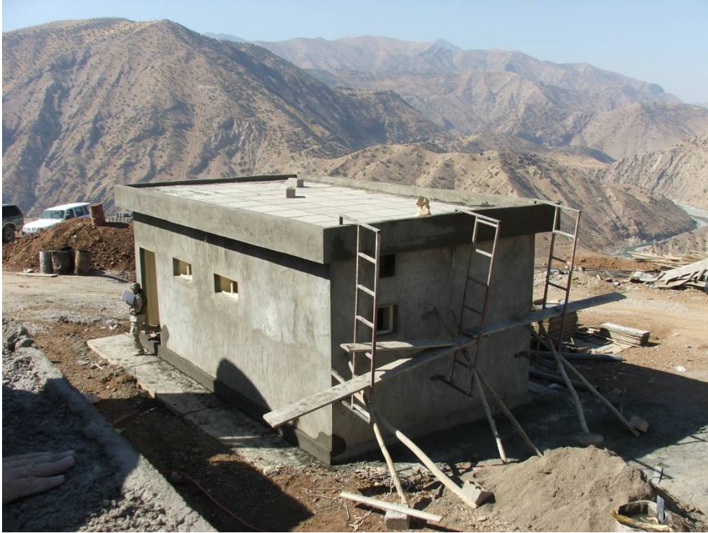
Site Photo 53. Exterior View of Jail Facility (Issawa #604 Border Post)
