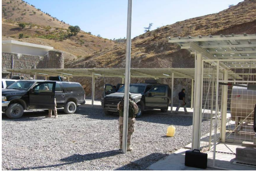
Site Photo 28. Automobile Covered Parking Area (Safrah #634 Border Post)
