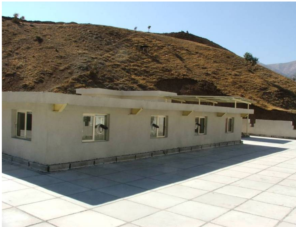
Site Photo 16. Exterior View of Atrium – Second Level (Safrah #634 Border Post)
