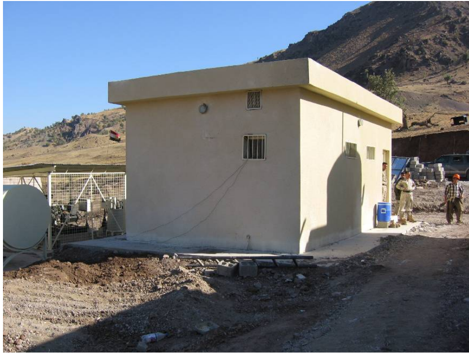
Site Photo 44. Exterior View of Jail Facility (Azmick #602 Border Post)
