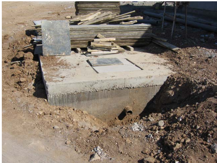
Site Photo 57. Septic Tank (Issawa #604 Border Post)
