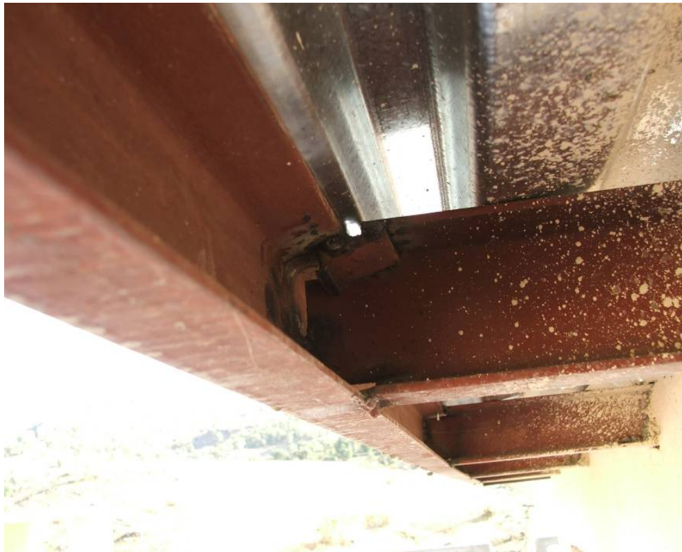
Site Photo 7. Channel Section to Channel Section Connection (Marwa #628 Border Post)
