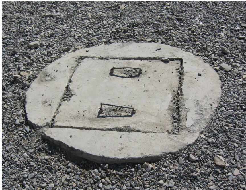
Site Photo 27. Access Hatch of Soakaway (Safrah #634 Border Post)
