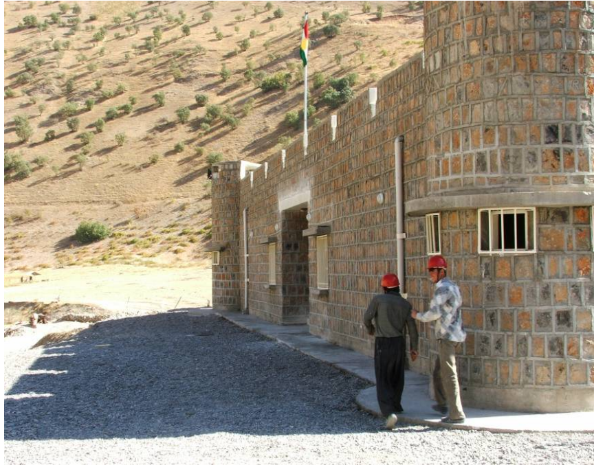
Site Photo 11: Exterior front view (Safrah #634 Border Post)
