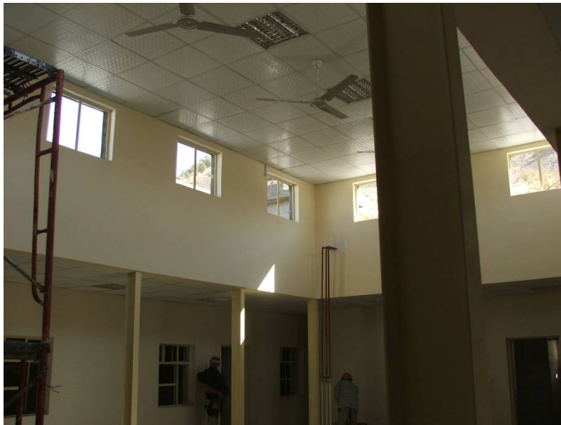
Site Photo 52. Interior Atrium (Issawa #604 Border Post)
