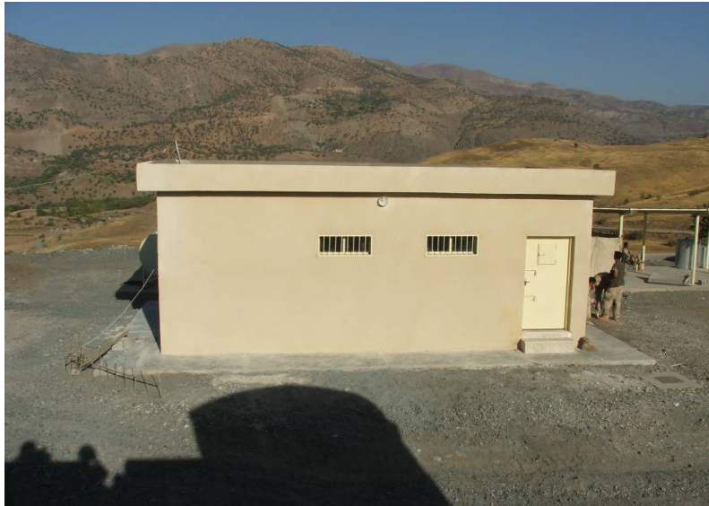
Site Photo 33. Exterior View of Holding Facility (Marwa #628 Border Post)
