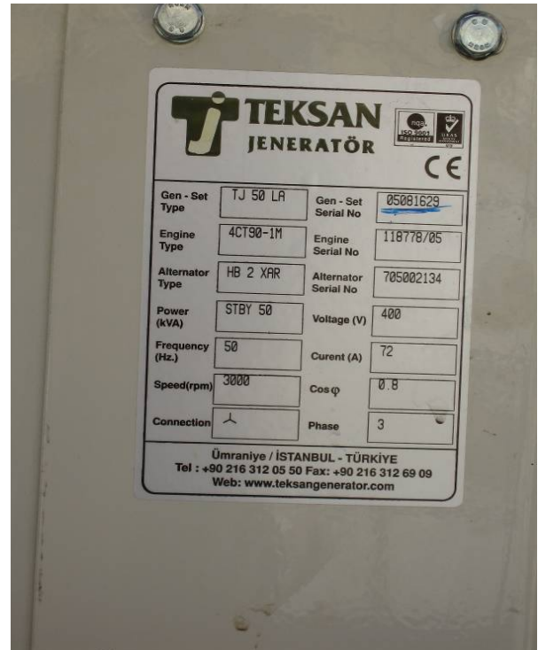
Site Photo 21 & 22. Generator Factory Nameplates (Safrah #634 Border Post)
