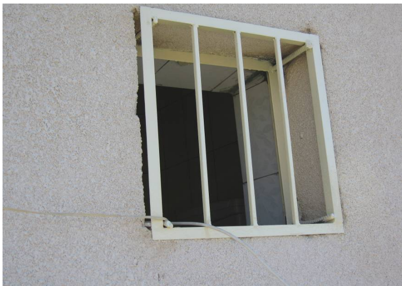
Site Photo 34. Metal Security Bars of Holding Facility (Marwa #628 Border Post)
