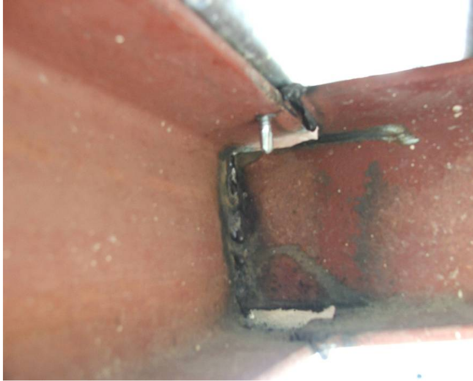
Site Photo 6. Channel Section to Channel Section Connection (Marwa #628 Border Post)
