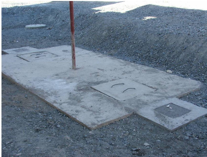
Site Photo 38. Septic Tank with Four Access Ports (Marwa #628 Border Post)
