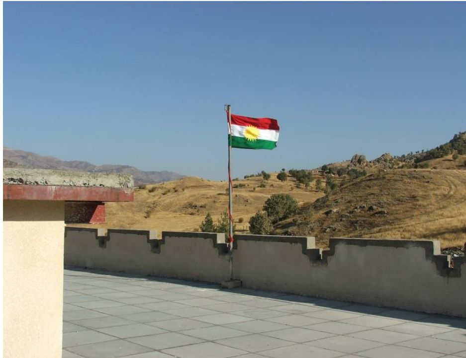
Site Photo 31. Roof, Parapet, and Flagpole (Marwa #628 Border Post)
