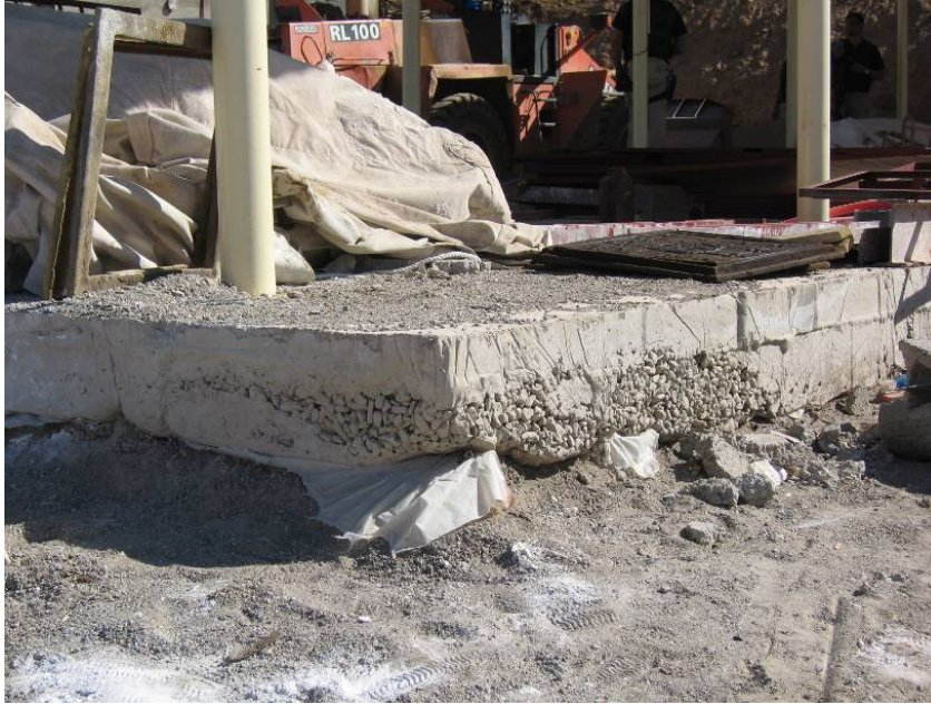
Site Photo 60. Concrete Pad of Automobile Parking Area (Issawa #604 Border Post)
