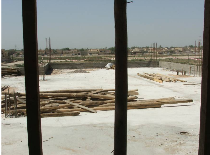
Site Photo 11. Ground Floor Roof Section
