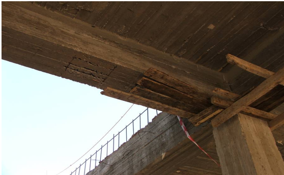
Site Photo 3. First Floor Ceiling Concrete Beam
