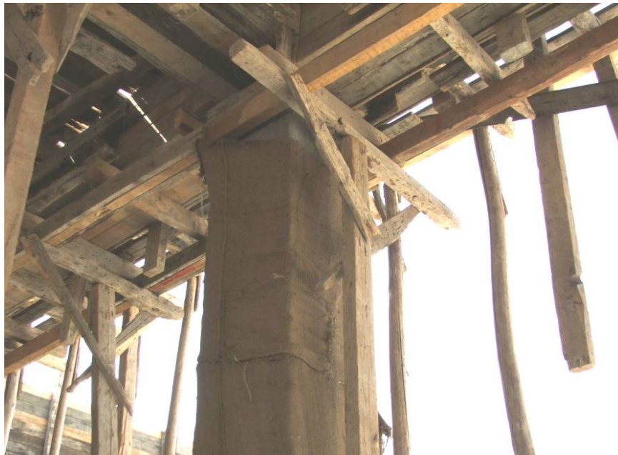
Site Photo 10. First Floor Column with Burlap Wrap
