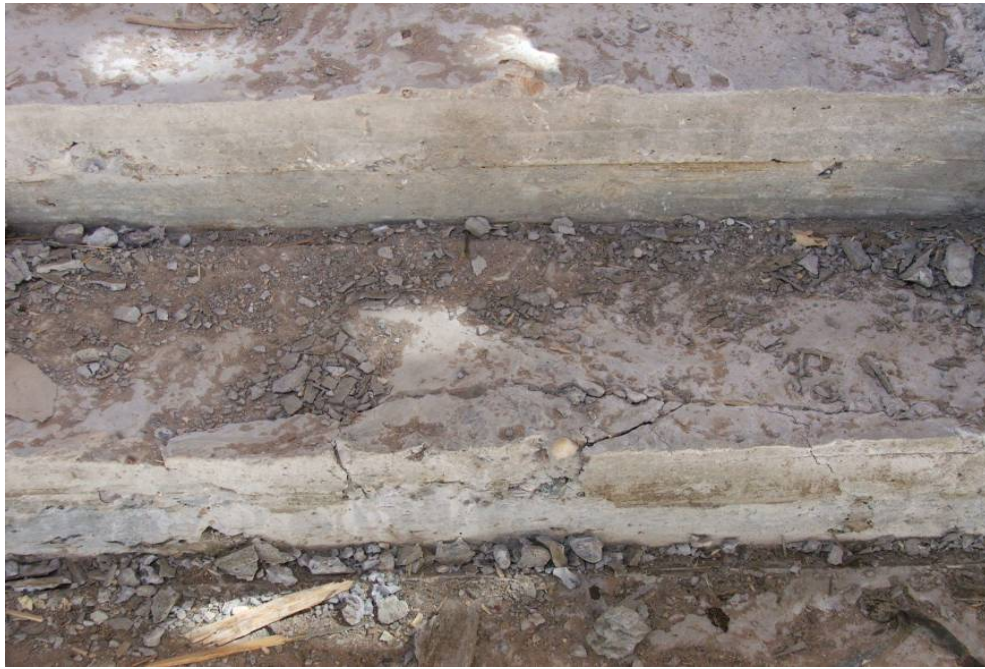
Site Photo 9. Ground Floor to First Floor Stairwell
