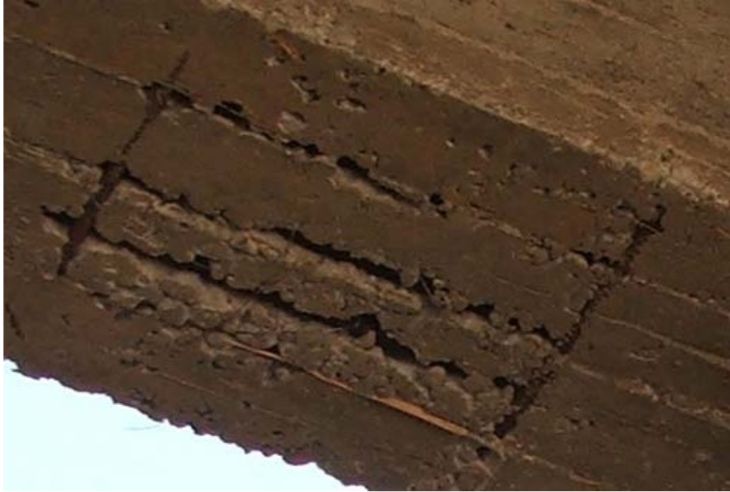
Site Photo 4. Close-Up View of Site Photo 3
