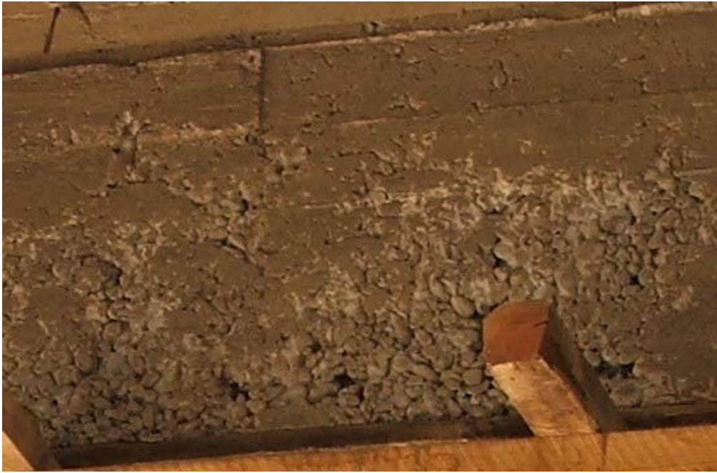
Site Photo 6. Close-Up of Site Photo 5
