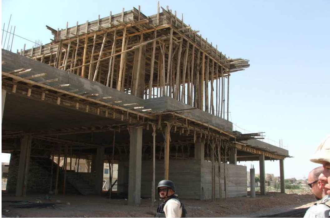
Site Photo 1. Ground Floor and First Floor Construction
