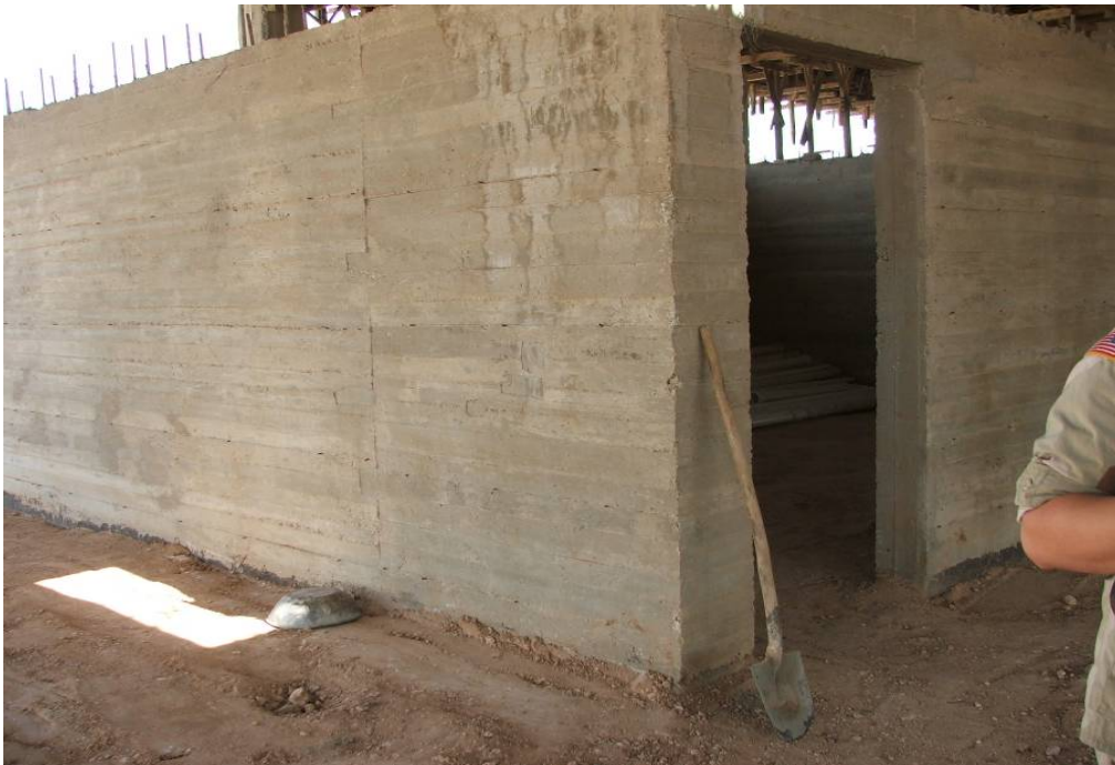
Site Photo 7. X-Ray Room Concrete Walls
