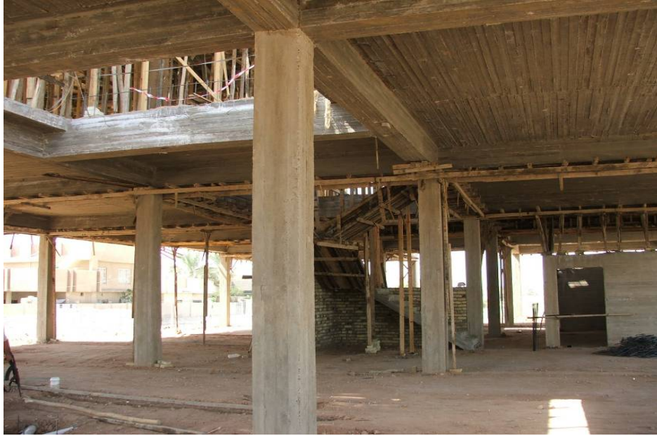
Site Photo 2. Interior Concrete Columns and Ground Floor Ceiling Slab
