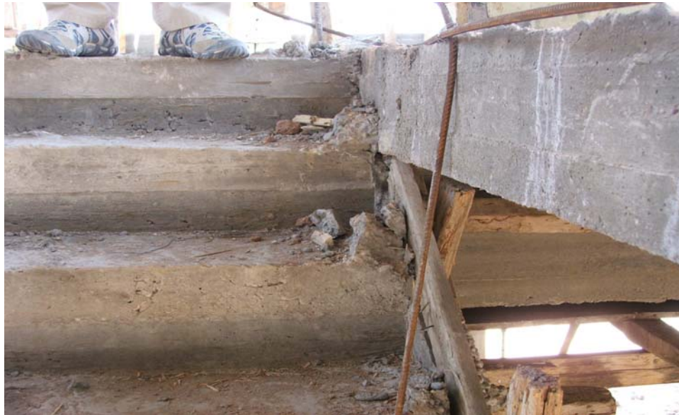
Site Photo 8. Ground Floor to First Floor Stairwell
