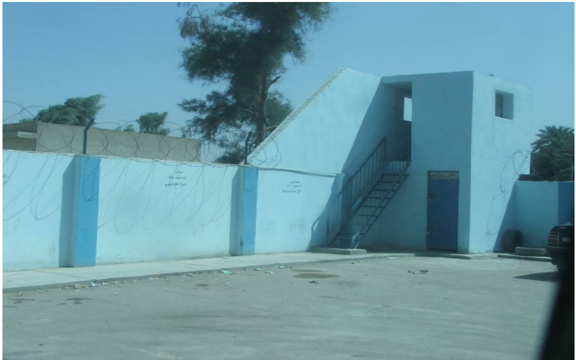
Site Photo 1. Guard Tower, Perimeter Wall with Concertina Wire on Top, Paved Parking Area, and Concrete Sidewalk
