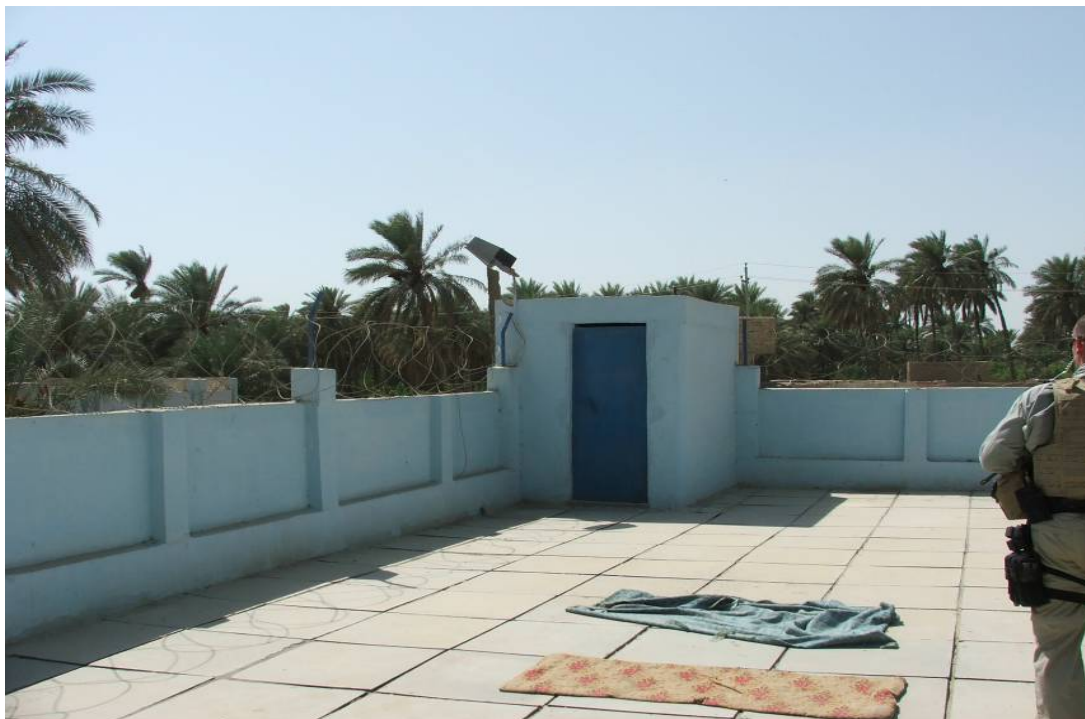
Site Photo 4. Tiled Roof
