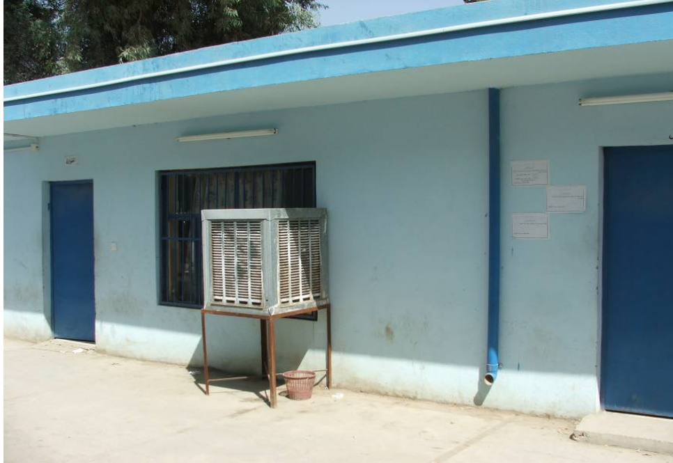
Site Photo 9. Exterior of the Three-Room Building
