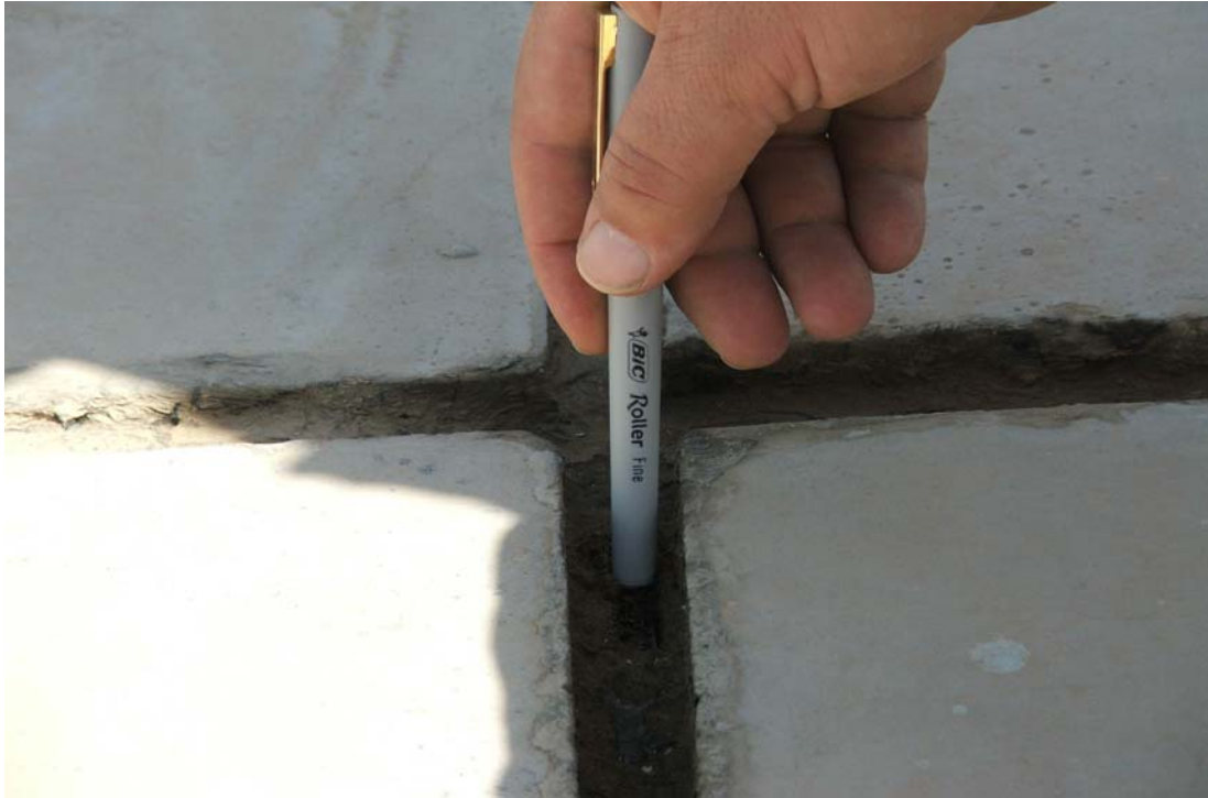
Site Photo 5. Mastic Seal between Concrete Roofing Tiles
