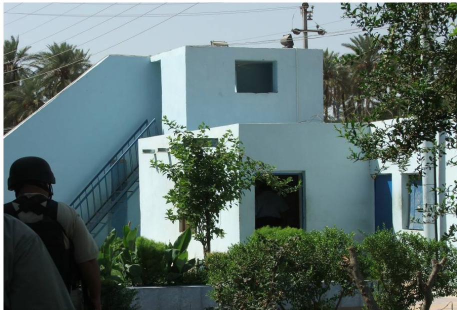
Site Photo 2. Corner Guard Tower (located near Front Entrance)
