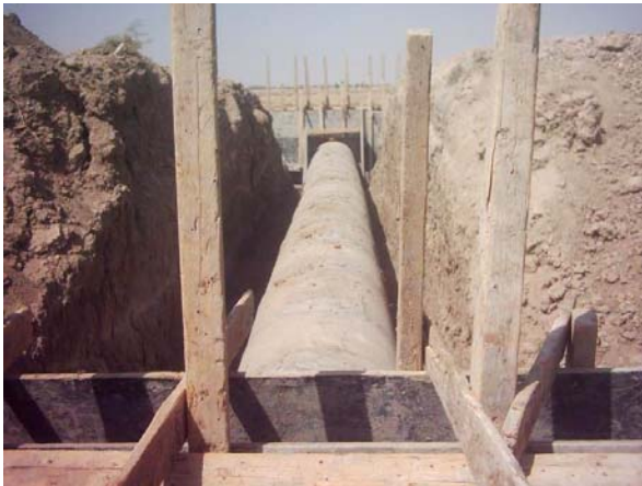
Site Photo 12. Pipe culvert in trench – Photo provided by USACE
