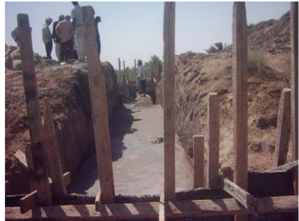
Site Photo 13. Pipe culvert encased in concrete – Photo provided by USACE
