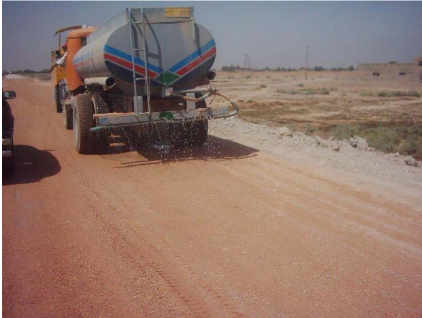
Site Photo 2. Water distributor adding moisture to the sub-base – Photo provided by USACE
