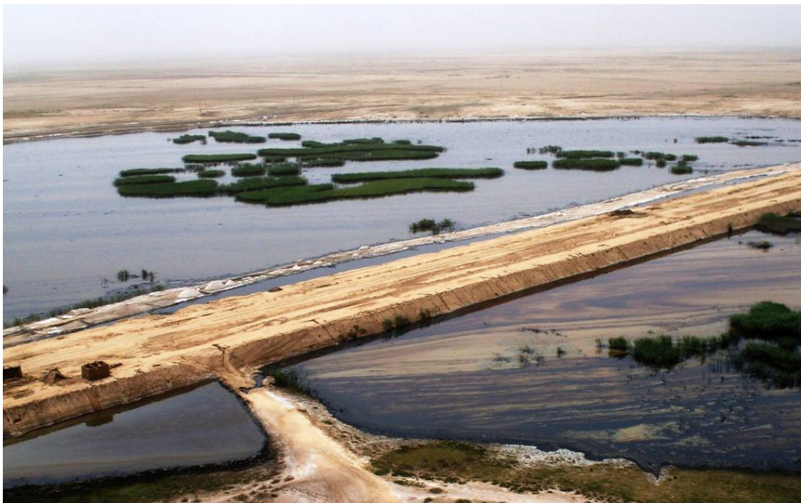
Site Photo 12. Aerial view of oil leakage along Kirkuk to Al Fatah Pipeline
