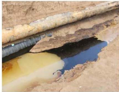
Site Photo 5. SIGIR Site Photo from February 2006. Oil Leakage from Existing Pipeline.
