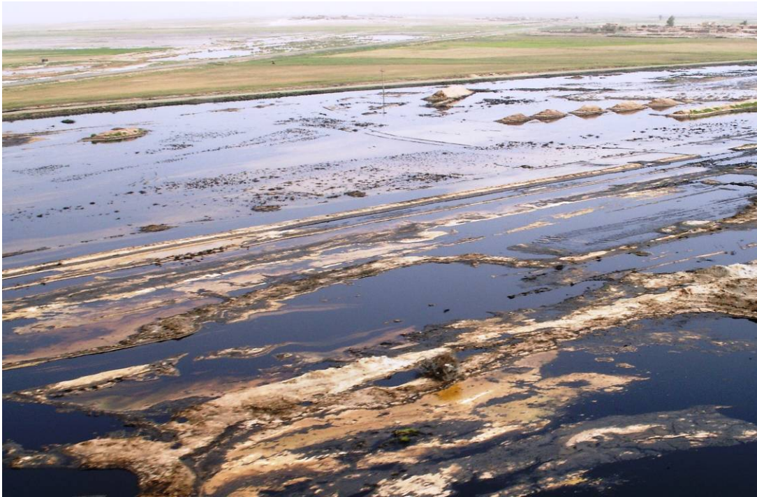
Site Photo 9. Aerial view of oil leakage along Kirkuk to Al Fatah Pipeline
