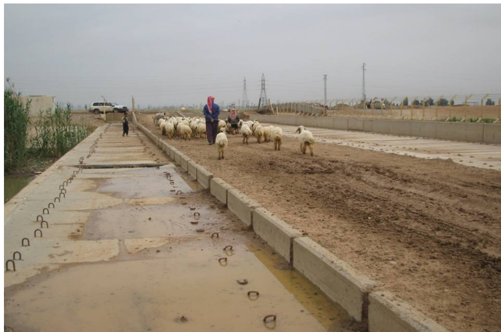
Site Photo 6. Photo of completed Kirkuk Irrigation Canal (Photo courtesy of PIJV)
