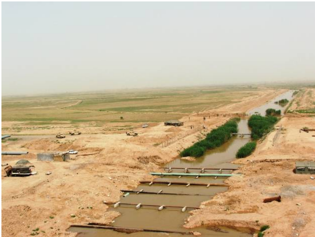
Site Photo 7. Aerial view of Zegeton Canal Crossing
