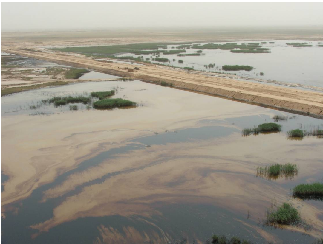
Site Photo 10. Aerial view of oil leakage along Kirkuk to Al Fatah Pipeline
