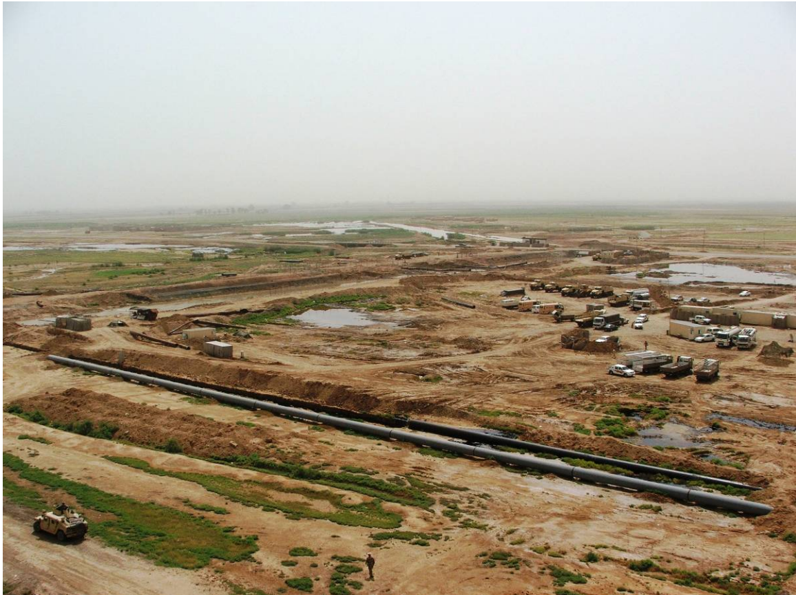
Site Photo 13. Welded pipe string at the Zegeton Canal
