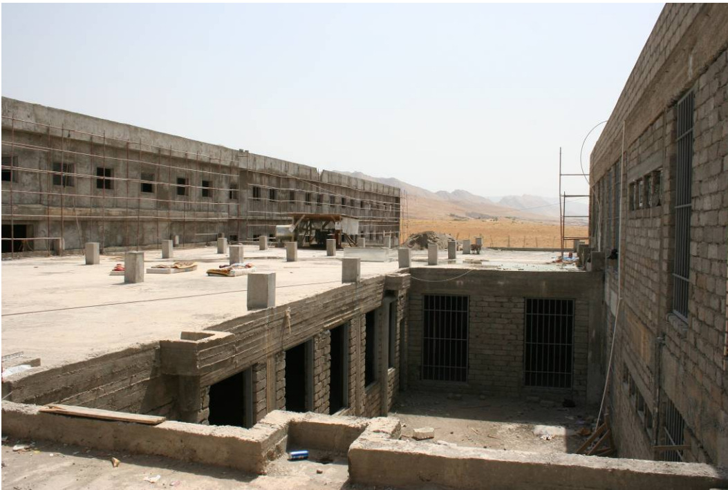
Site Photo 12. Left side of photo shows completed exterior finish work, while right side shows an unfinished wall.
