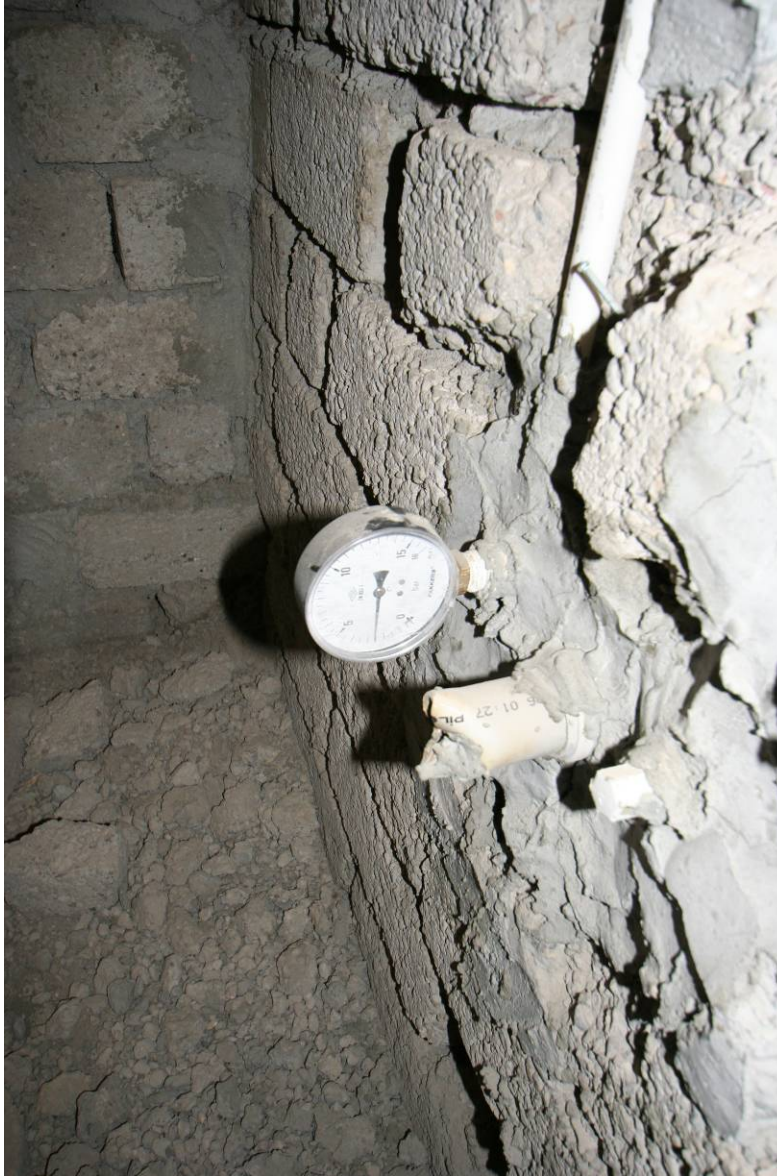
Site Photo 18. Domestic water line pressure test was in progress.
