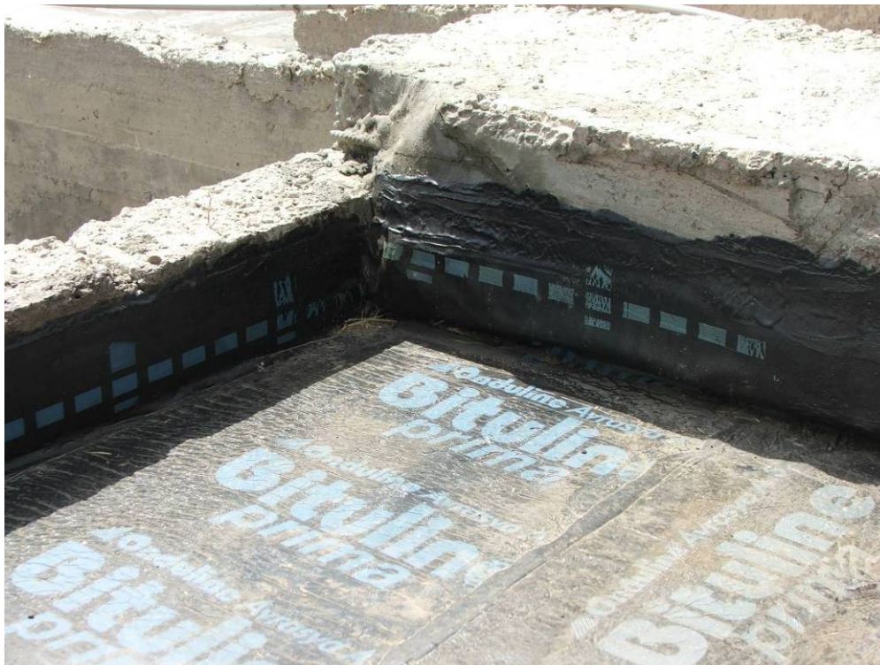
Site Photo 3. Bituminous waterproofing membrane.
