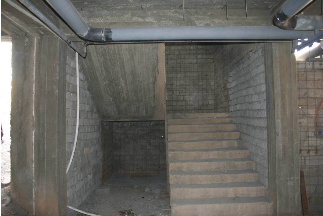
Site Photo 8. Pre-finish front view of poured concrete stairs.
