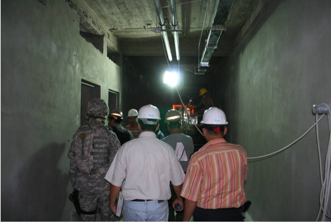
Site Photo 11. Concrete finished interior walls.
