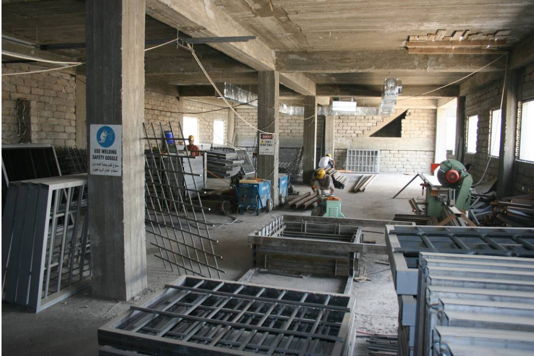
Site Photo 5. Pre-fabrication shop for security protection bar assemblies.
