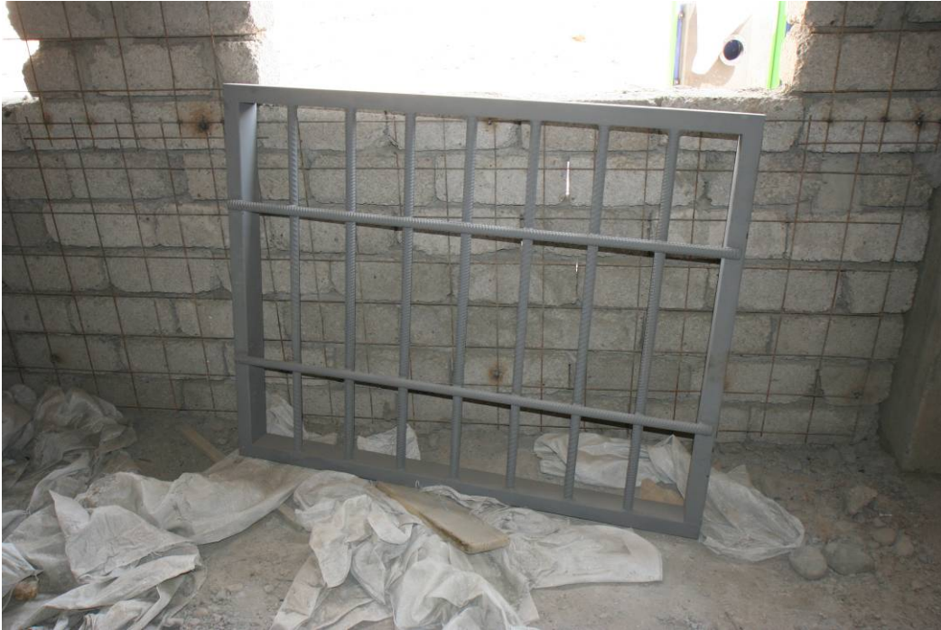
Site Photo 7. Pre-fabricated security protection bar assembly staged for installation.
