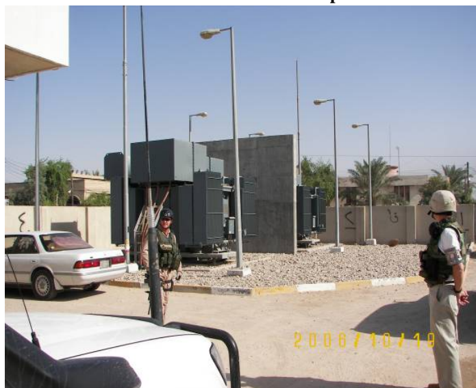
Site Photo 3. Al Seraji substation view of internal walls
