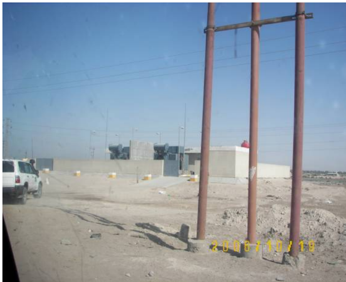
Site Photo 2. Al Hamdan substation perimeter walls
