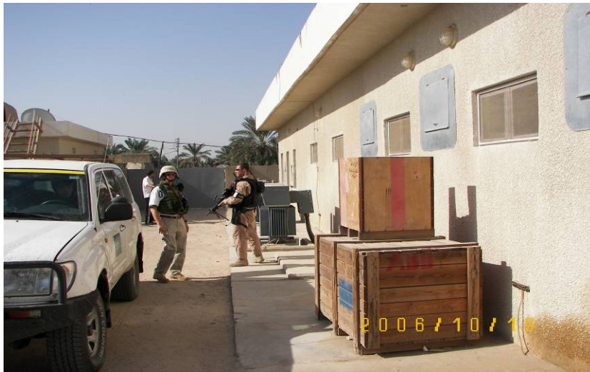
Site photo 12. Boxes thought to contain the spare parts delivered to the Al Seraji substation
