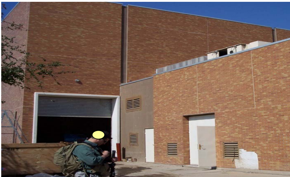
Site Photo 1. Sadr City Al Qana'at raw water pump station.
