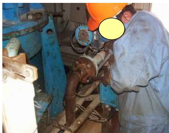
Site Photo 6. Rehabilitating pumps. (Picture courtesy of USACE)
