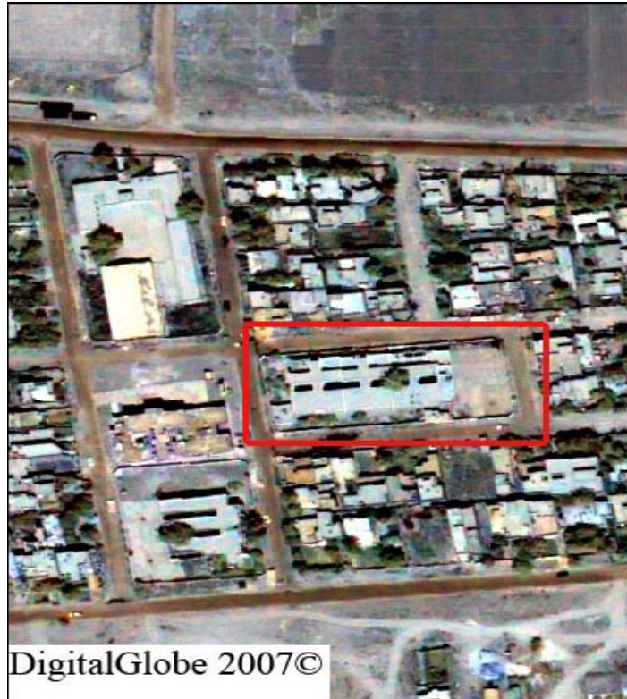
Aerial Image 1. Imagery overview of the Al Escandrona School taken on 16 September 2007.
