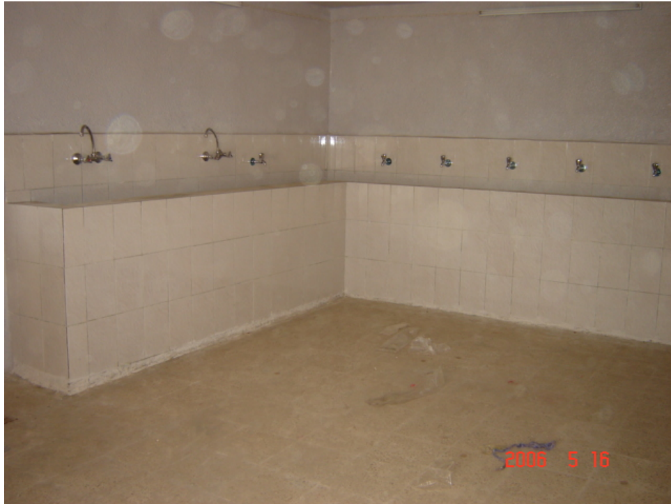
Site Photo 6. Sinks after renovation (Photo courtesy of USACE)
