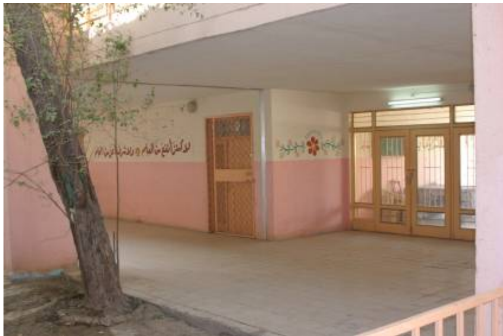
Site Photo 12. Interior painting after occupancy and use (Photo courtesy of USACE)
