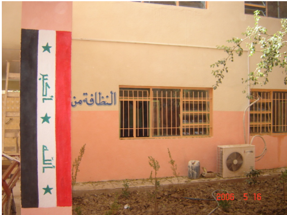
Site Photo 5. Exterior painting after renovation (Photo courtesy of USACE)
