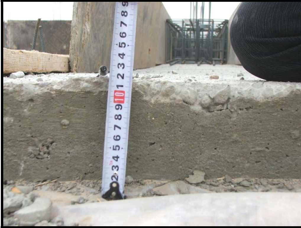
Site Photo 19. Blind (lean non-structural) concrete was sufficiently thick throughout facility.
