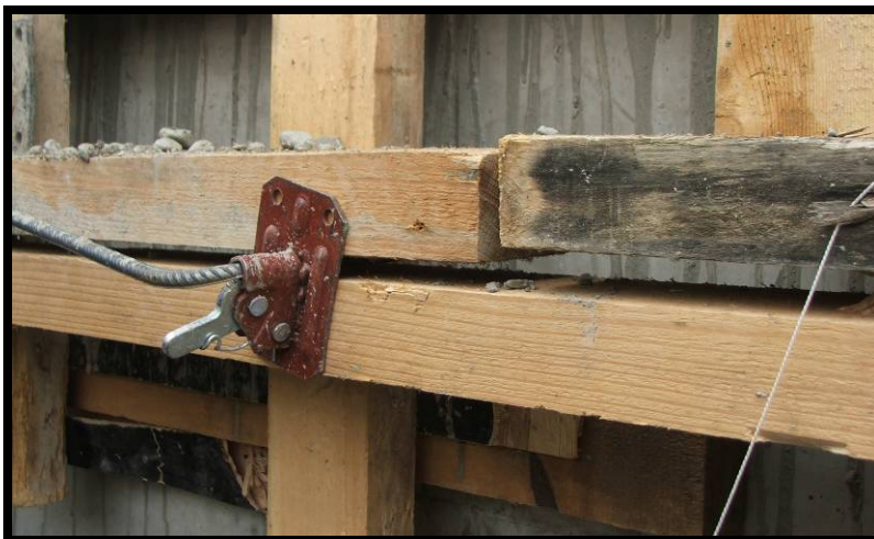
Site Photo 17. Locks effectively controlled form movement during casting.
