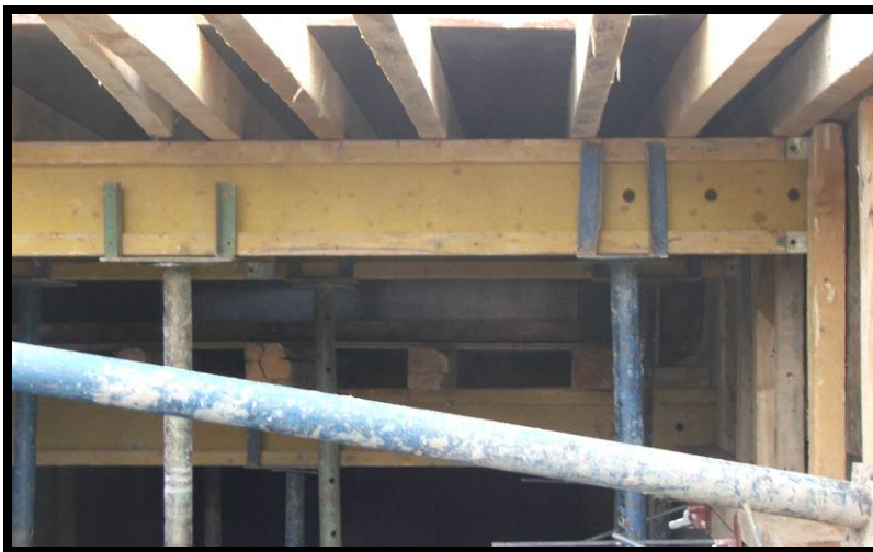
Site Photo 16. Throughout facility, form work was excellent.
