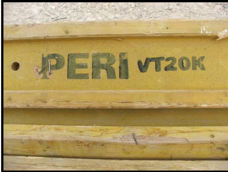
Site Photo 14. Per Scope of Work, a manufactured form girder system was used.
