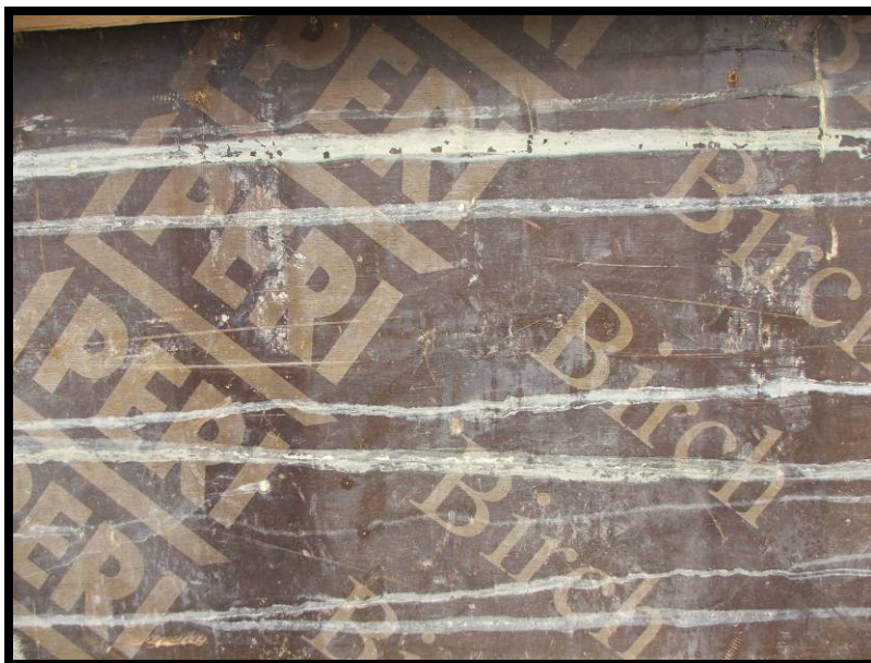
Site Photo 15. Contractor used premium forming materials.
