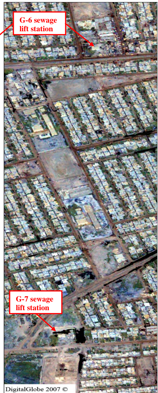
Aerial Image 2. Location of the Al Ghazaliyah G-6 and G-7 sewage lift stations
