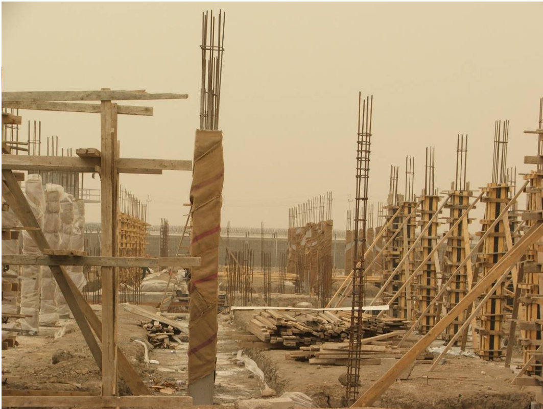
Site Photo 3. Concrete column with burlap for curing
