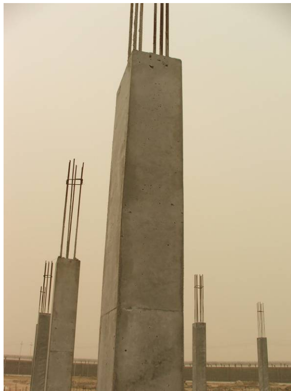
Site Photo 2. Concrete columns
