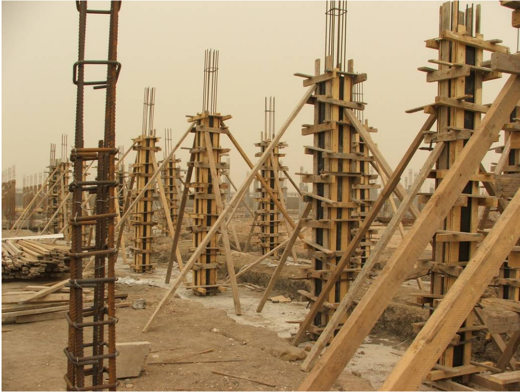
Site Photo 1. Ongoing construction work for the concrete frame and foundations
