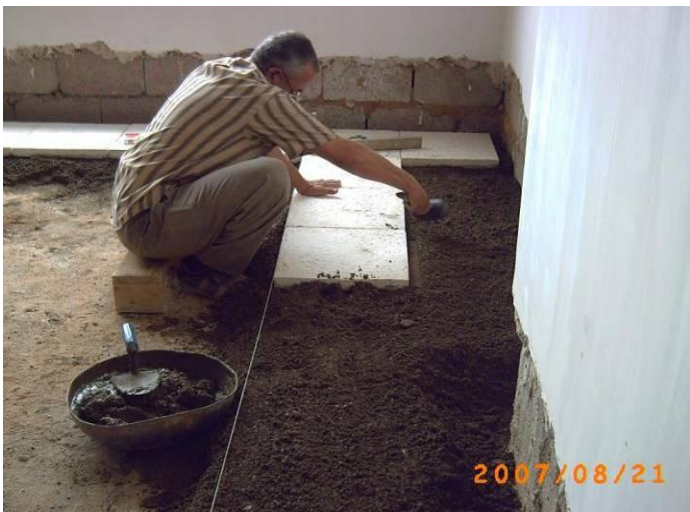
Site Photo 4. Tile placement (Courtesy of GRC)
