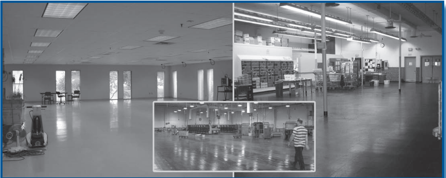
Audits of facility optimization showed, that while the Postal Service has made progress in optimizing its existing space, it can do more to dispose of excess interior space in a more timely manner. Pictured: West Edina Carrier Annex, Minneapolis, MN (left), Marysville, CA P&DF (center), South Eastern Station (right).
