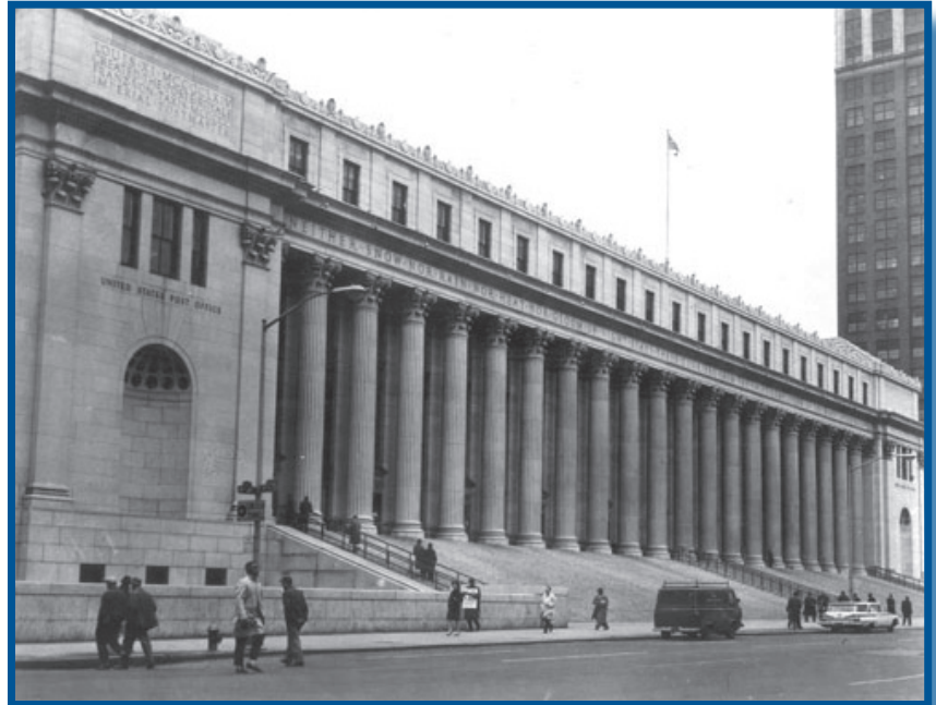
The OIG audits postal retail units — post offices, stations and branches — to determine whether they comply with nine key financial reporting controls.
