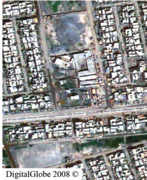
Aerial imagery of the Al-Ghazaliyah G-6 Sewage Lift Station.
