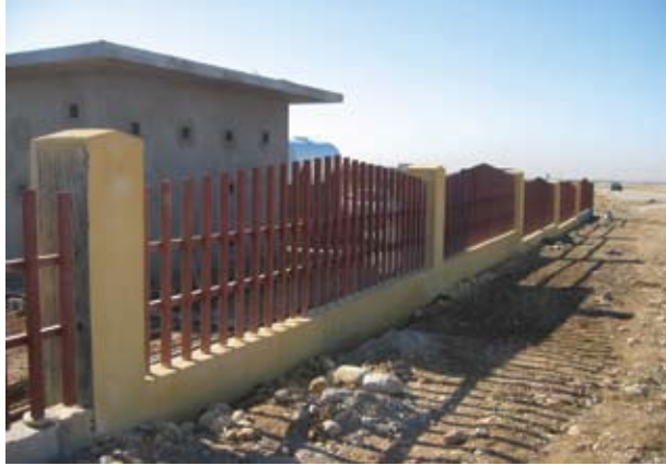
Perimeter fence segment.
