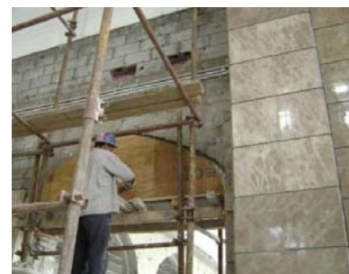
Main entrance stone-cladding work. March 2008.
