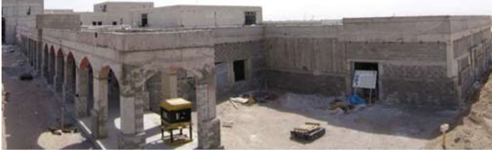
Corner view of the Basrah Children's Hospital. March 2008.
