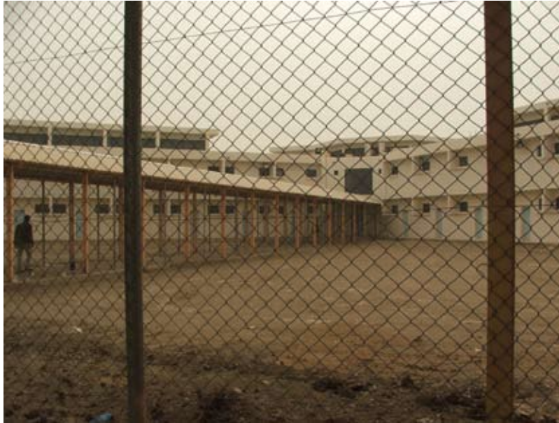
Entrance and walkway of inmate housing.
