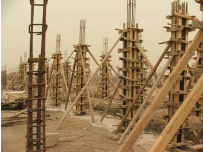
Ongoing construction work for the concrete frame and foundations.
