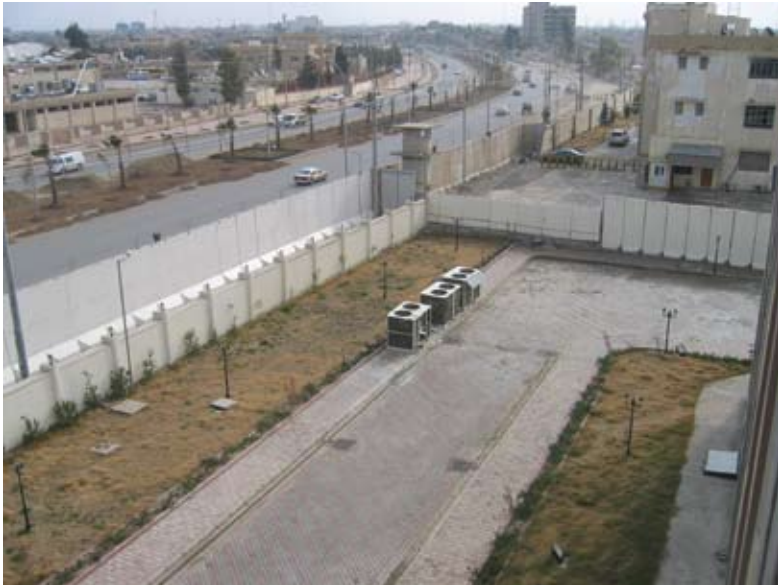
Repaired wall, installed T-walls, and reconstructed guard shack. Photo taken from the roof of the services building.
