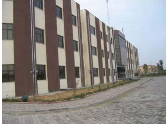
Refurbished services building.
