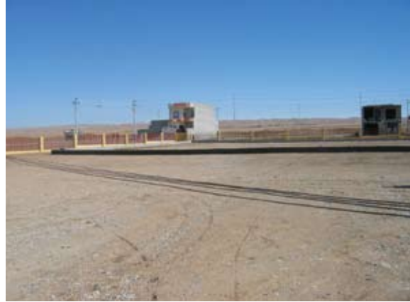
Graded facility grounds.
