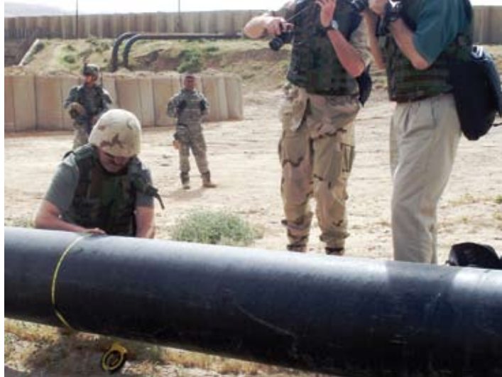
SIGIR Inspection team examining the oil pipeline at Al Fatah.
