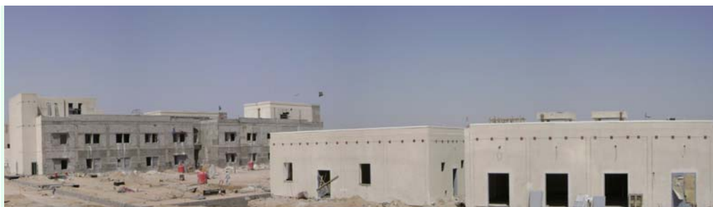
Basrah Children's Hospital—Main and ancillary hospital buildings. March 2008.
