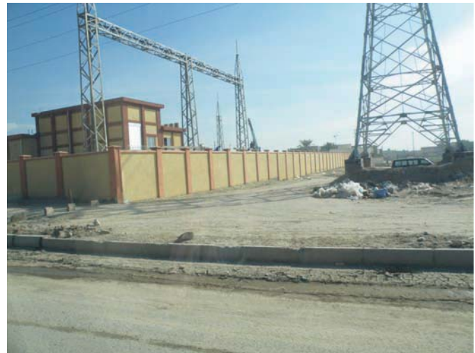
Exterior perimeter wall.
