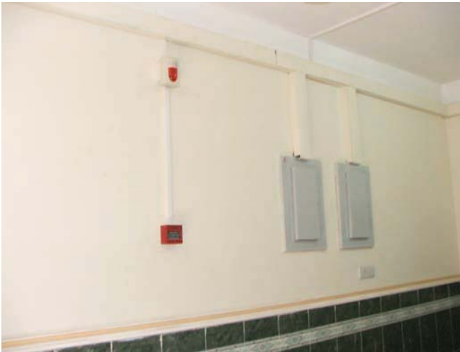
Installation of new wire molding, outlets, and new main distribution panels.
