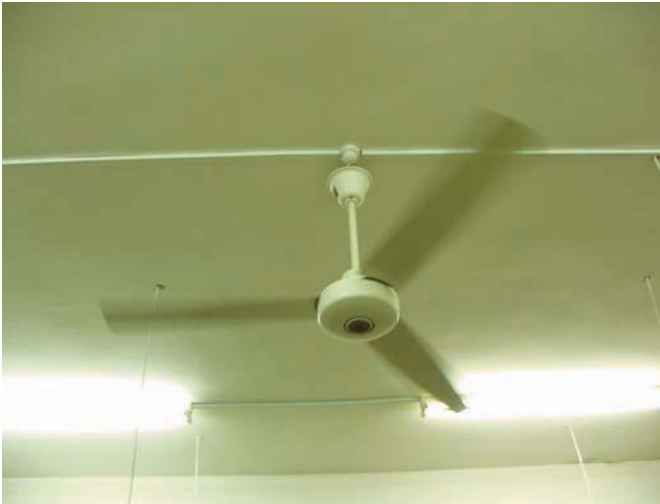
Interior of the hospital administration building.
