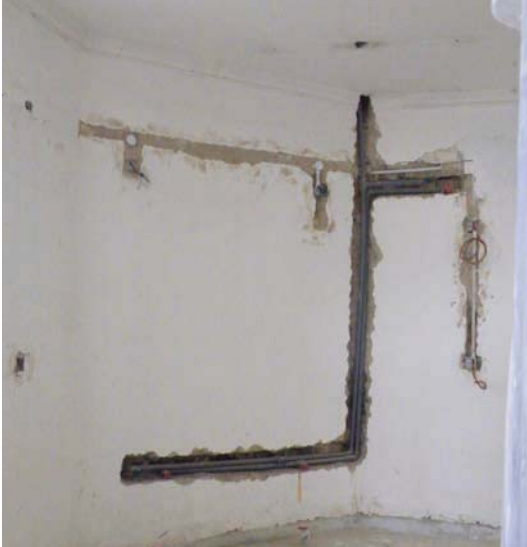
Partially completed interior finishing.
