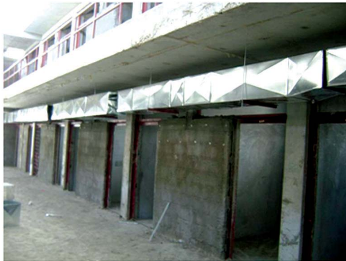
A new cellblock erected at Nassriya prison. (OPA photo)
