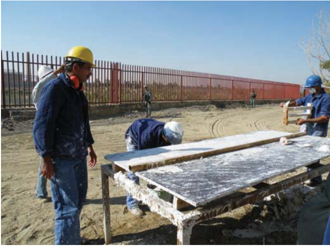
Contractors pouring molding for future installation.
