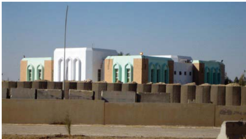
Courthouse in Anah, Iraq, rebuilt with assistance from Coalition forces. (DoS photo)
