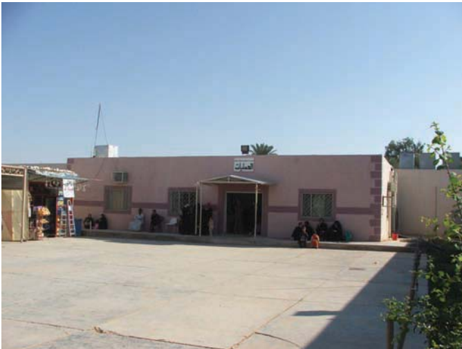
Exterior of the surgery wing building.
