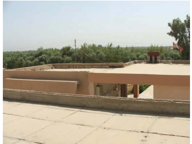
Roof tiles after renovation.
