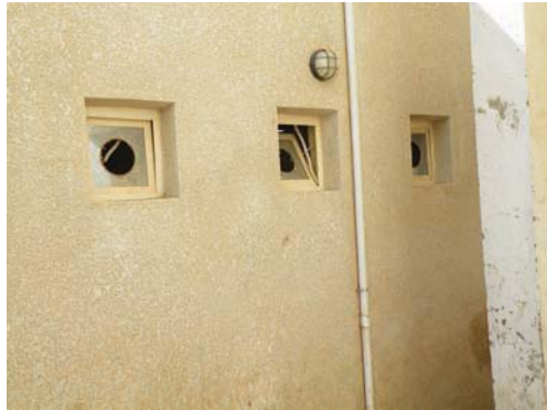
Exhaust fans removed from latrine buildings.
