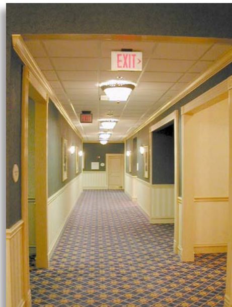
The walls and ceiling of this means of egress must meet specific flame spread rating standards.
